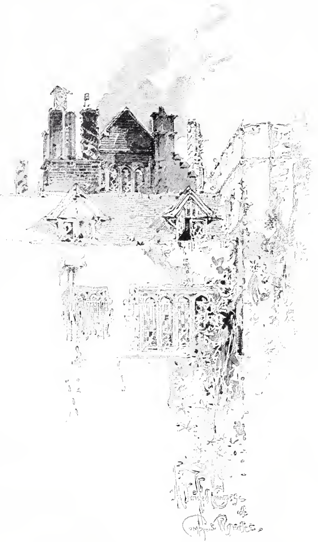
THE TWISTED CHIMNEYS, COMPTON WYNYATES.
