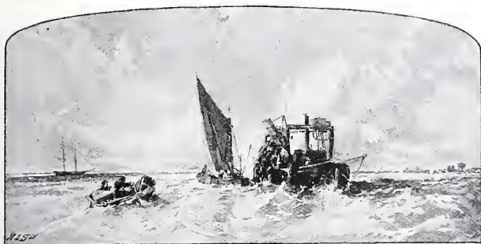
DREDGING ON THE MEDWAY.
