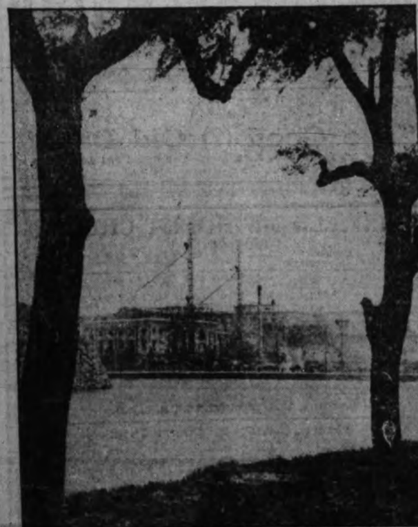
CONCRETE MIXERS ROAR —In sharp contrast to the quiet of the Palace grounds is the feverish activity across the Moat. The whirr of electric hoists and roar of concrete mixers is heard everywhere. The building under construction in the centre is the Imperial Theatre.
