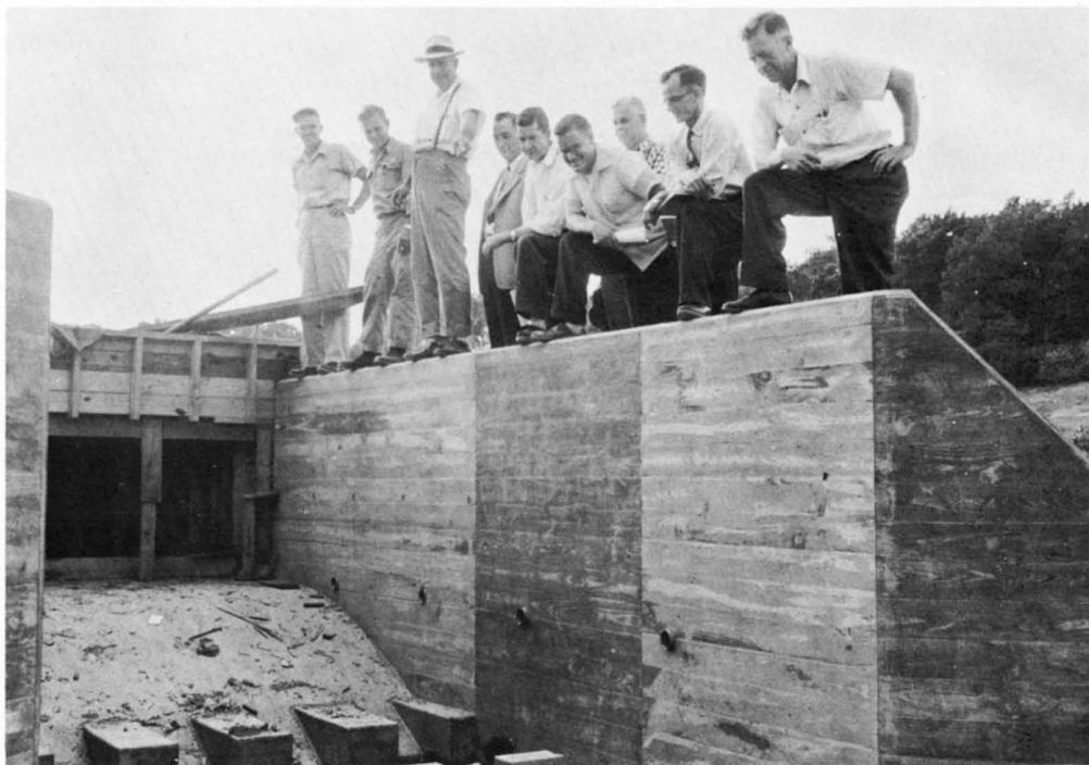
As the watershed-protection program of the Upper Hocking got underway, farmers and businessmen took an active interest in the work. Here a group is inspecting the concrete dissipator blocks used in the outlet of the first dam to be constructed. Crop inlets, of concrete, provide for a slow, uniform passage of runoff waters into the channel below. The concrete work is finished before the embankment or earth fill is constructed to form the dam.
