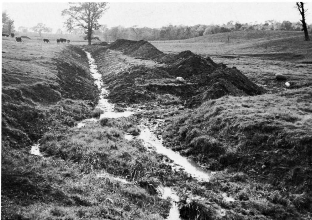
Work to conserve soil and water on the farms in the watershed has been carried out simultaneously with flood-prevention measures. One practice was to make open drains to eliminate soggy meadows and increase production. Outlets provide safe methods of water disposal for the field waterways. Waterways were graded into former gullies and natural water courses. Grassed waterways are left as a permanent protection to the land and are not plowed during cultivation of fields.
