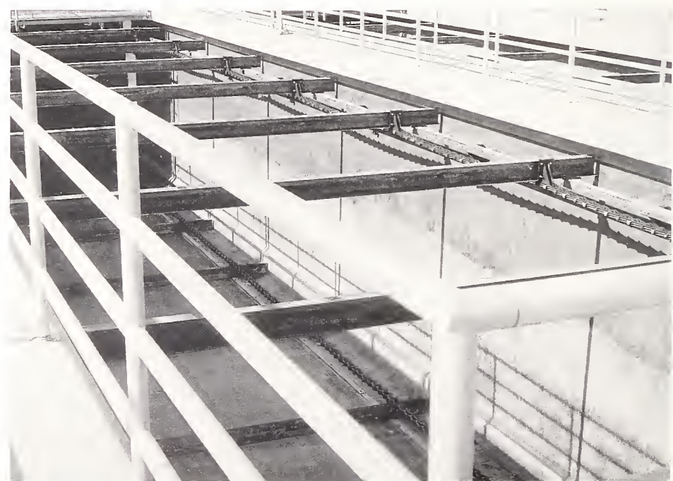
Figure 5.6. Undamaged clarifier tank at the Tillman Water Reclamation Plant.
