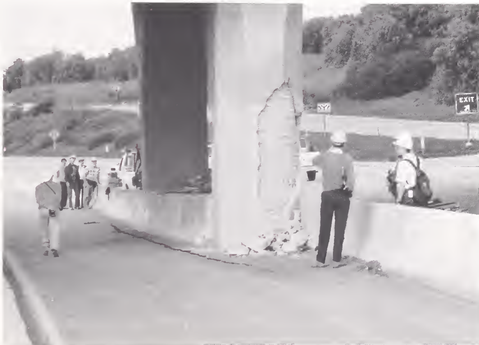
Figure 4.31. SR118 Ruffner Ave. Overcrossing, easternmost central pier, looking to the west.
