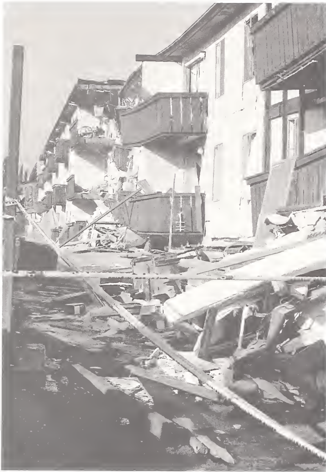
Figure 3.4. At the Northridge Meadows apartment complex near the epicenter the first story in several of the buildings collapsed, killing sixteen people. The second and third stories remained essentially intact. Large portions of the first story in these buildings were open space for parking. This type of collapse occurred in a significant number of similar apartment buildings throughout the affected area.
