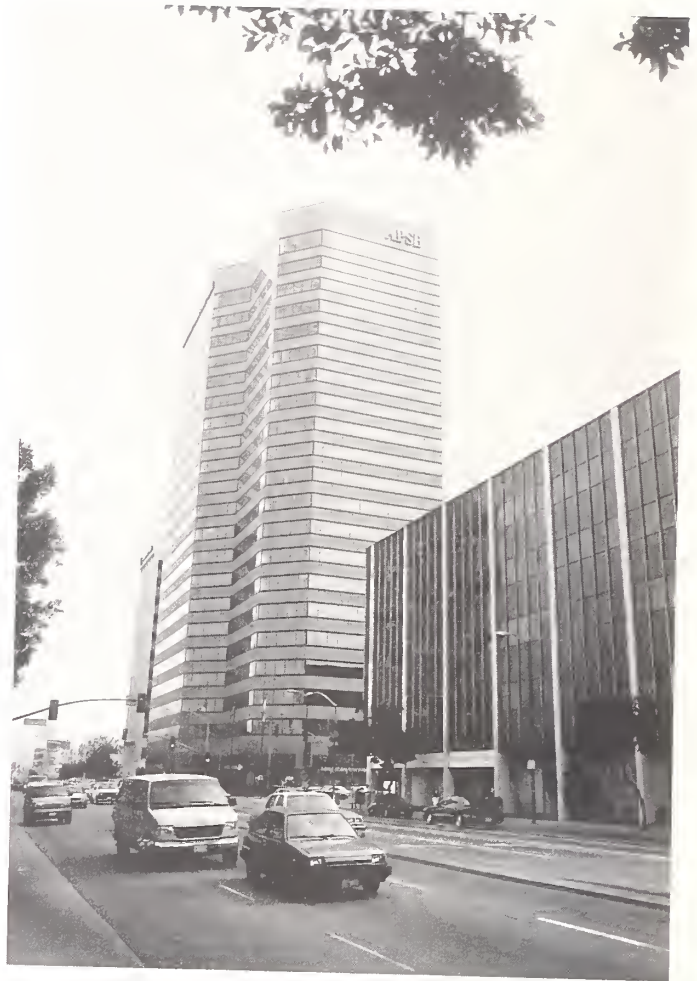
Figure 3.57. There was no evidence of damage to the 22-story American Pacific State Bank in Sherman Oaks. The adjacent eight-story parking garage had damaged columns.
