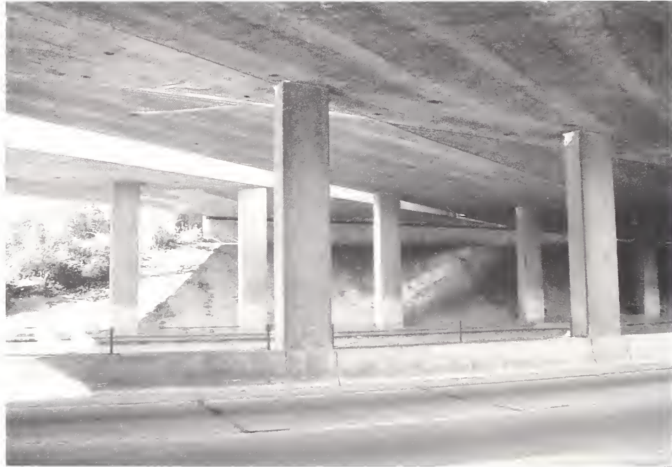
Figure 4.47. Eastbound lane of Ventura Freeway as seen from the northbound lane of Hollywood Freeway.
