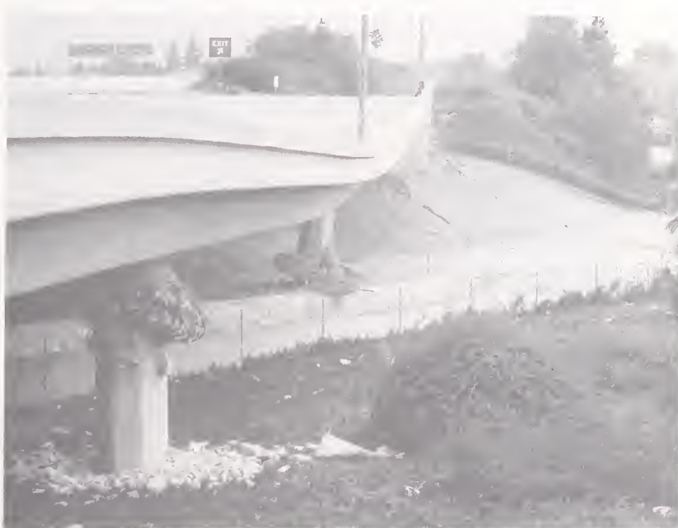
Figure 4.26. Ground-level view of State Route 118 at Bull Creek Canyon Channel, looking along the south edge, towards the east.
