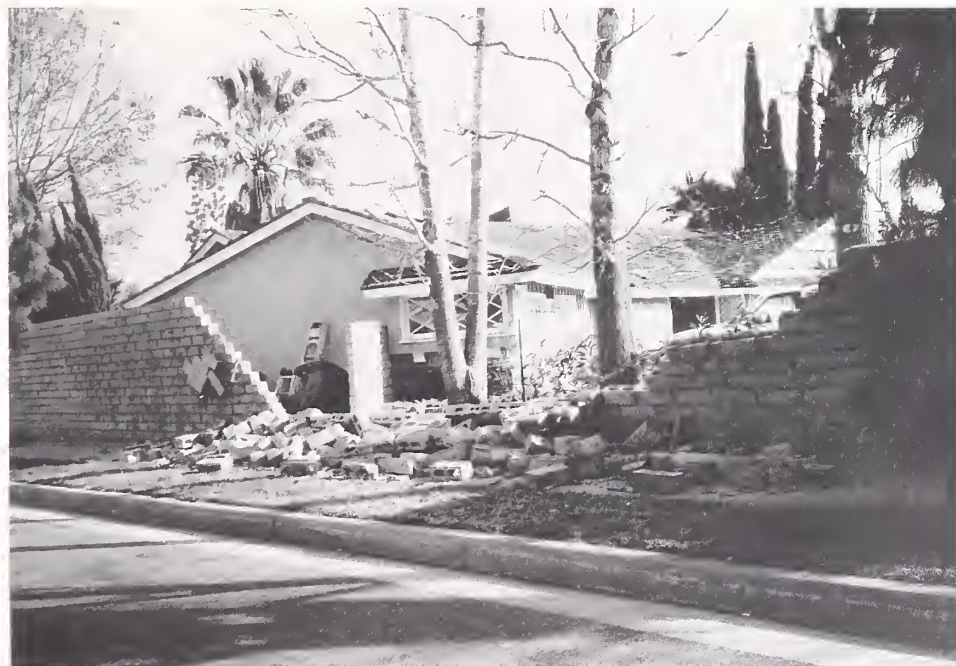
Figure 3.18. Damage to masonry privacy fences was ubiquitous. Many of these fences were tall enough to have been a serious threat to passersby when they failed. Luckily, due to the early morning hour of the quake, yards and sidewalks were essentially deserted.
