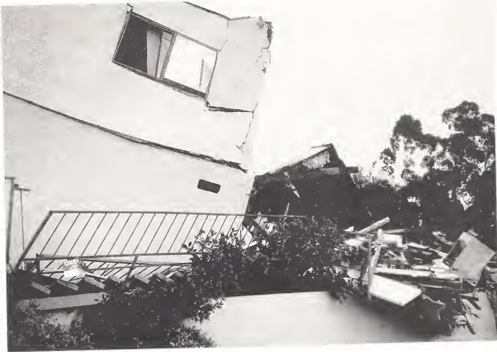
Figure 6.4. Partially collapsed apartment building with fire damage in the rear.
