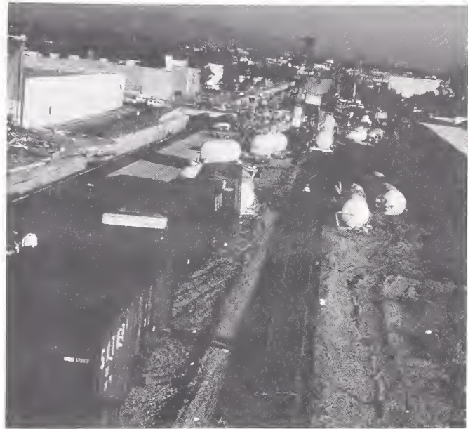
Figure 5.18. Derailment of a 64-car freight train in Northridge. The incident resulted in the spill of 30 000 L of sulfuric acid and 7500 L of diesel fuel. (Photo courtesy of LeVal Lund.)
