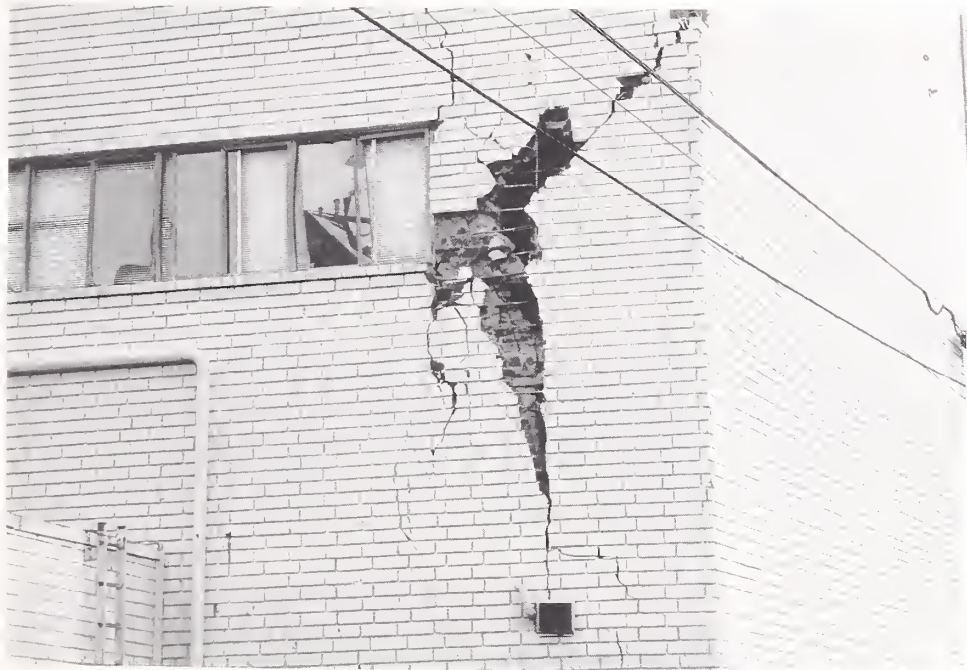
Figure 3.59. A close-up view of the damage shows the pattern of reinforcing used in the masonry facade.
