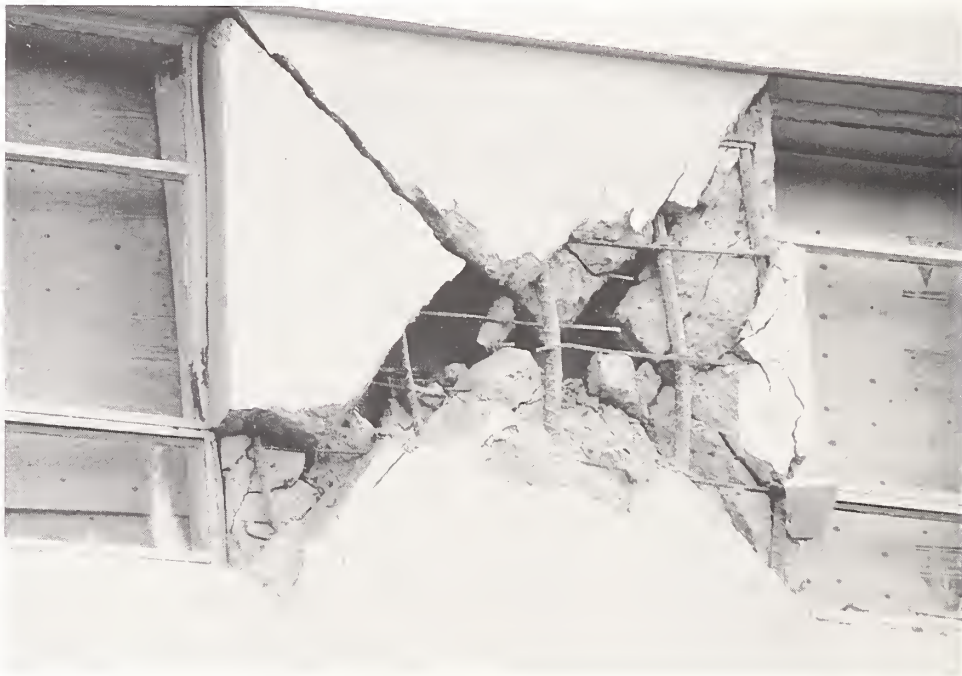
Figure 3.24. The transverse reinforcement in the St. John's hospital window piers was spaced at about 150-200 mm on center with 90° hooks at the ends, typical for construction of its age (about 50 years old).
