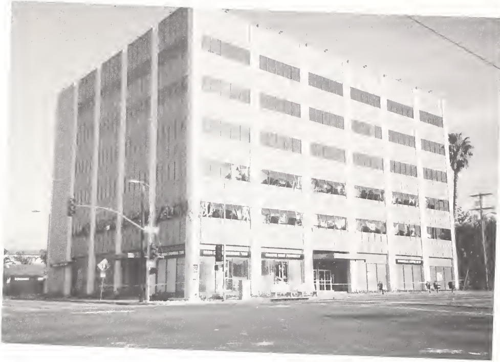
Figure 3.45. The six-story L-shaped concrete-frame Barrington Building on Olympic Boulevard in West Los Angeles lost its vertical-load carrying capacity at the second story.
