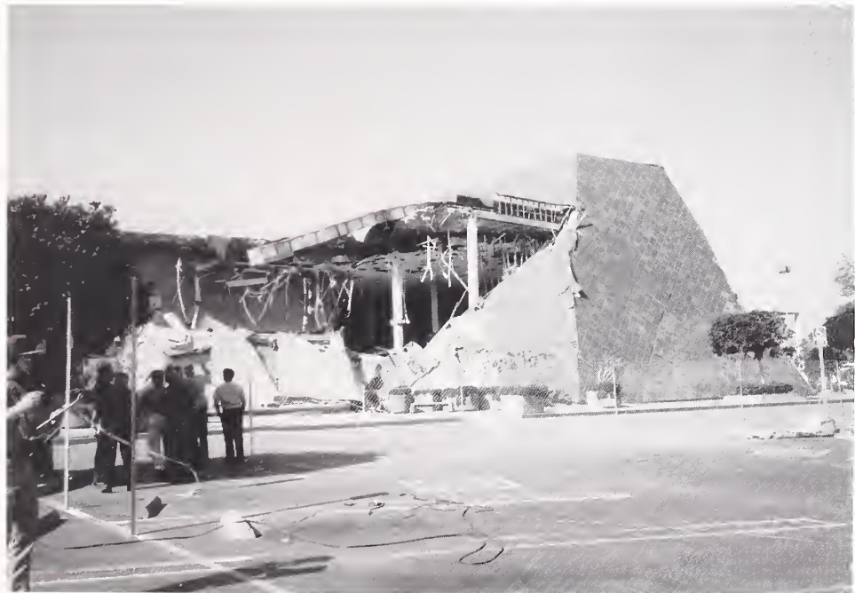
Figure 3.30. The Bullock's department store had an extremely irregular vertical geometry. At the northeast end it was shaped like a truncated pyramid.
