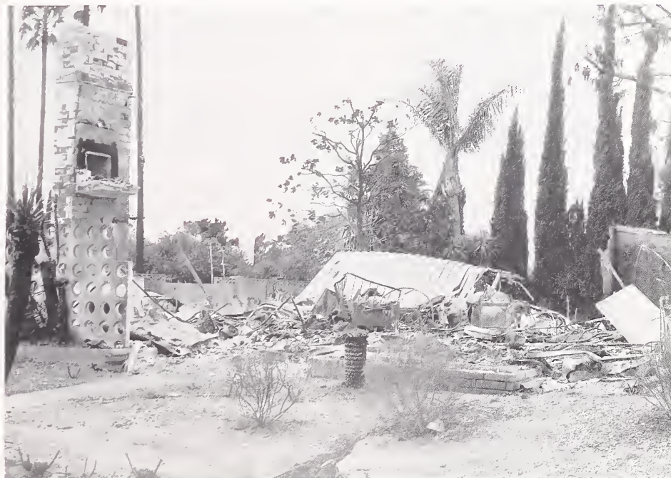
Figure 5.12. Houses destroyed by a fire resulting from the rupture of the 0.6-m gas main along Balboa Boulevard.
