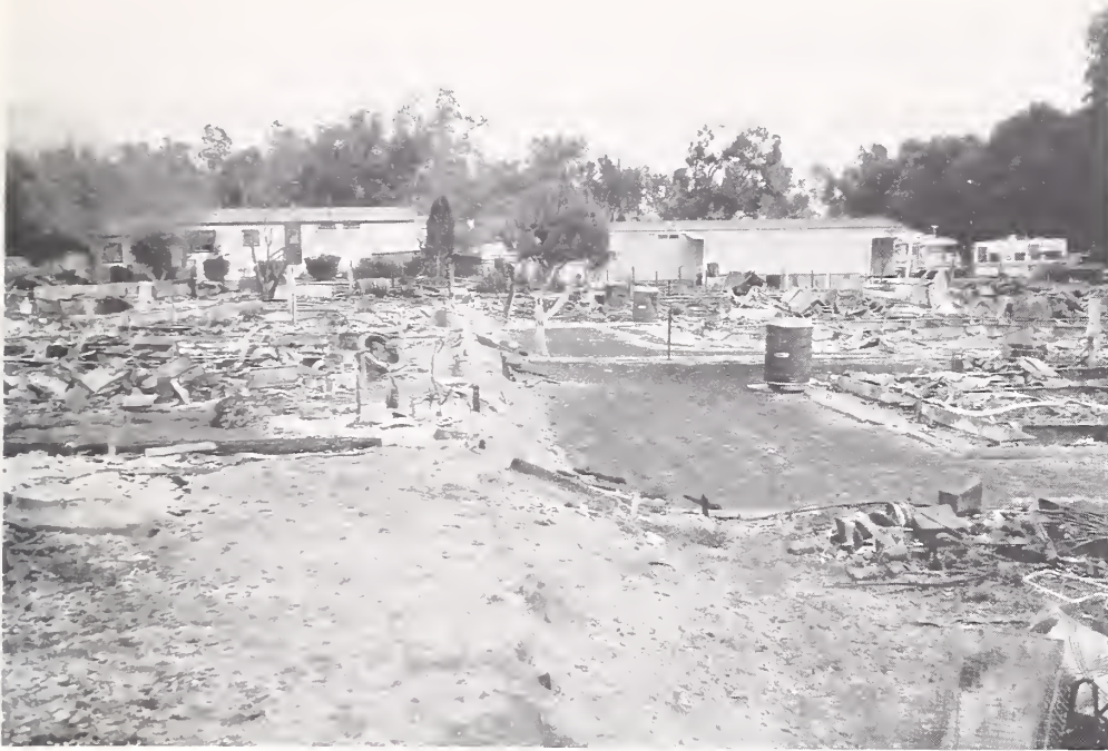
Figure 6.9. Impact of a multiple unit fire in a manufactured housing development.
