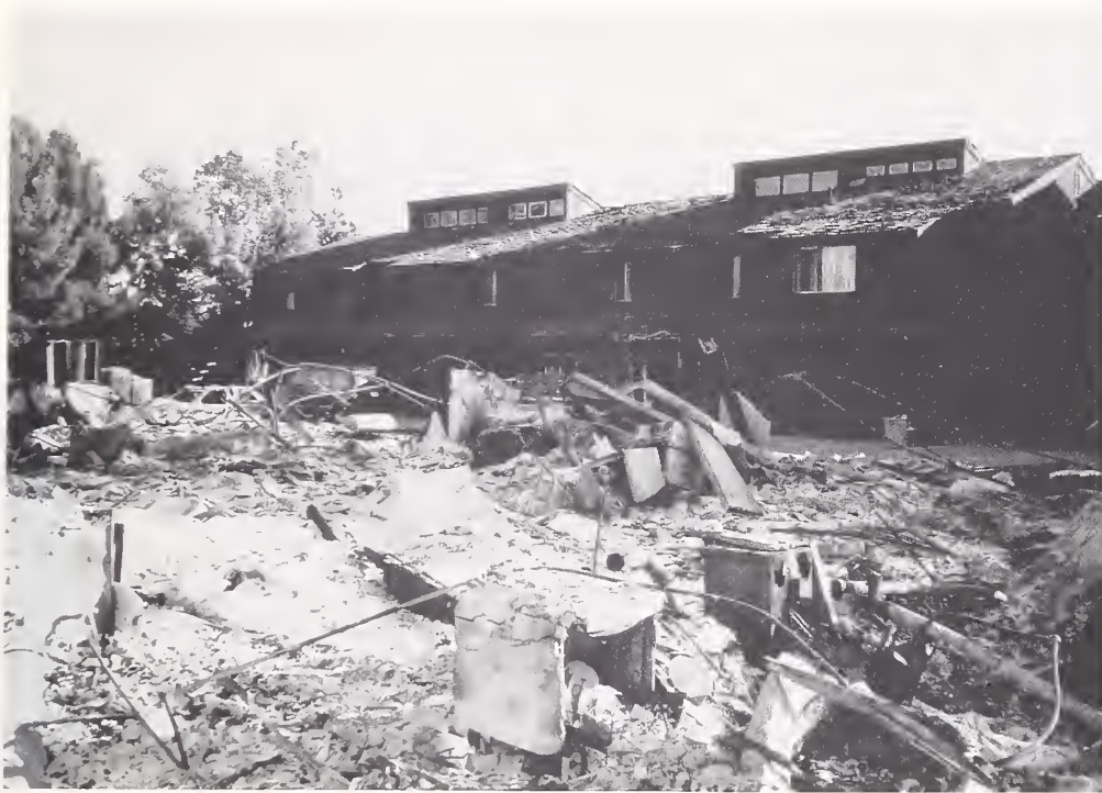
Figure 6.6. Multi-family residential building destroyed by fire.
