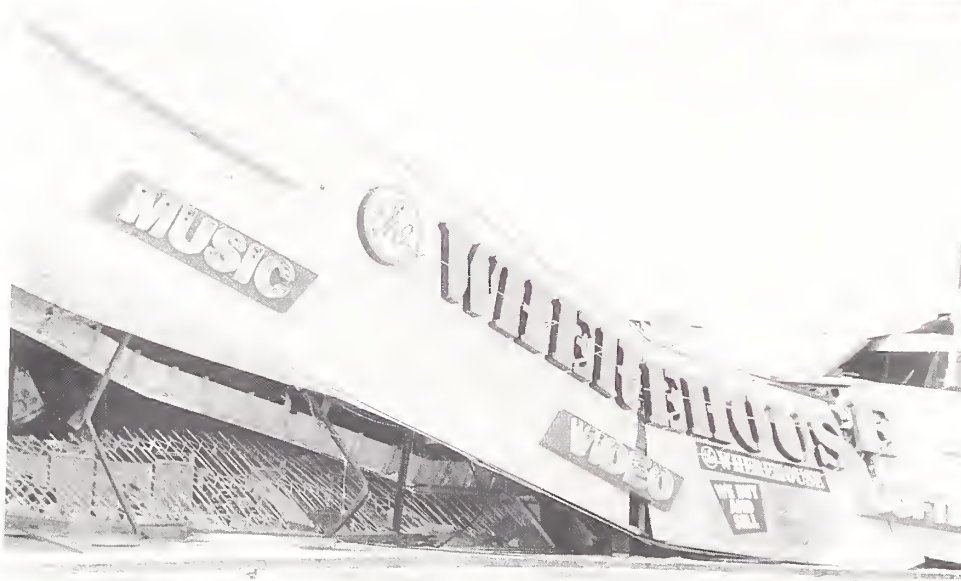
Figure 3.32. Many commercial buildings were damaged in the blocks south of the Northridge Fashion Center. The single-story Warehouse collapsed completely.
