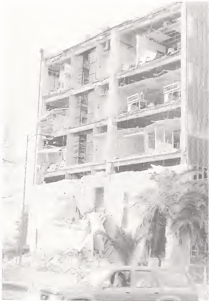
Figure 3.49. The east end wall and stair tower of a five-story apparently steel-framed office building on Sherman Way in Reseda collapsed. The enclosing masonry wall became detached from the structure and slid to the ground, with the upper stories remaining intact. The doorway opening in the wall, shown here resting at about the second story level, originally provided access from the top story to the stair tower.
