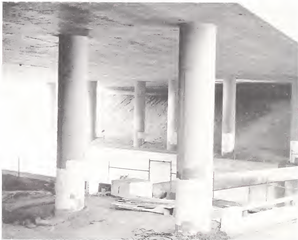
Figure 4.33. I10 Bridge over Ballona Creek, looking to the southwest.
