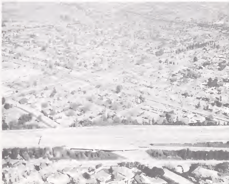
Figure 4.25. Aerial view of State Route 118 at Bull Creek Canyon Channel, looking to the north (Photo courtesy of FHWA).
