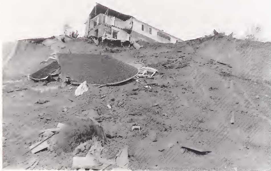
Figure 2.8. A landslide along the Pacific Coast Highway north of Santa Monica undermined the foundation of a house at the crest of the slope, bringing a portion of the house down.
