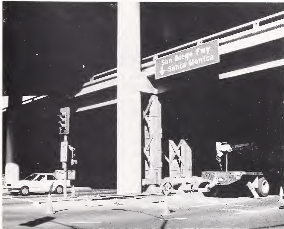
Figure 4.53. Overview of the outrigger joint at the SR90/I405 interchange, Jefferson Boulevard Undercrossing, center bent, west side, looking to the north.
