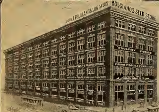
GENERAL OFFICES AND STORES PRATT, LIGHT, & ELLICOTT STS.
