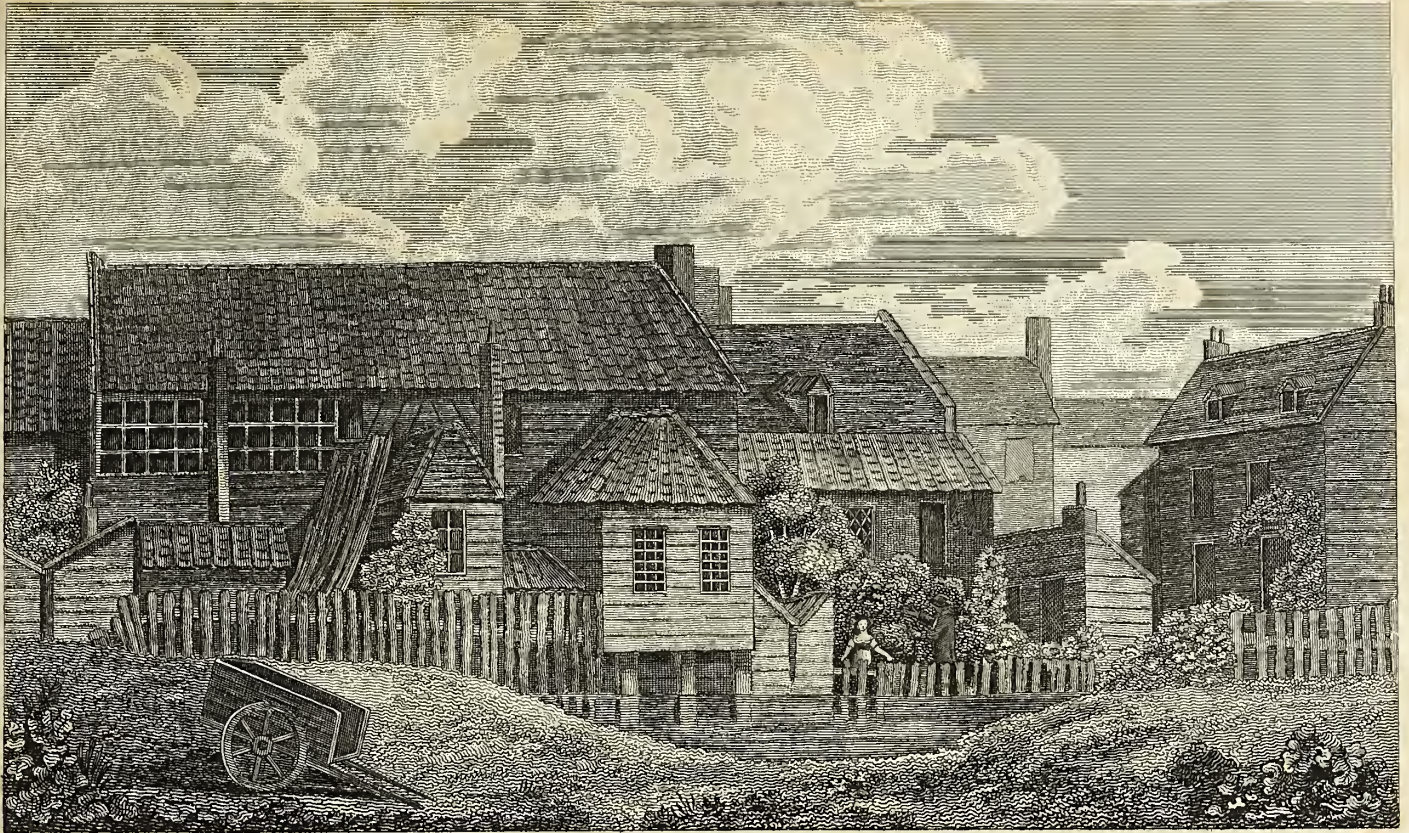
John Bunyan's Meeting-house, Loar-street, Gravel-lane, Southwark.
