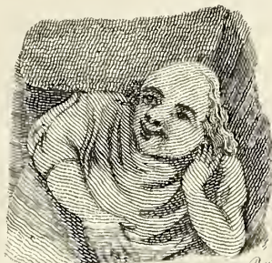
Head which supports a large Beam in the Chamber under the Roof at the east end, near Henry VII's Chapel.
