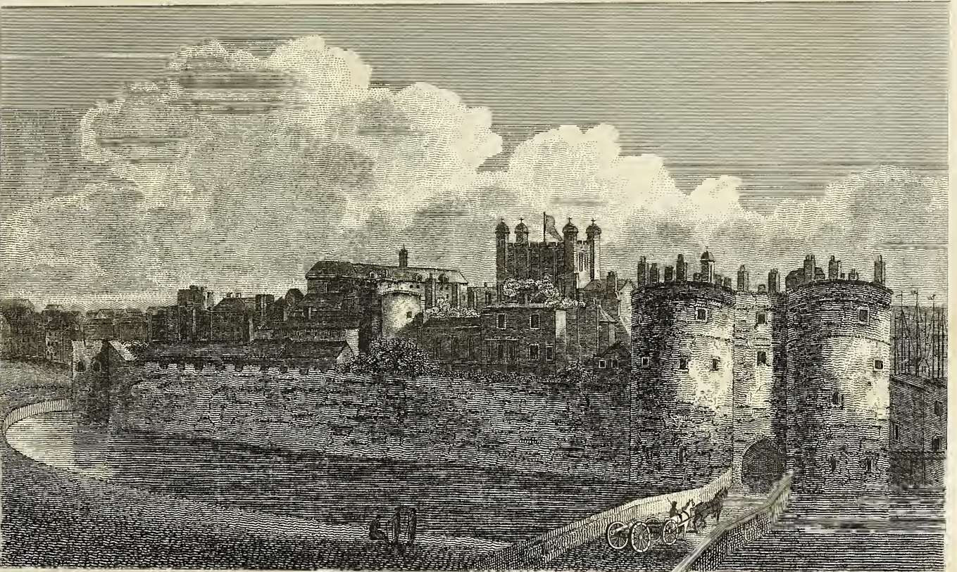
View of the Tower.
