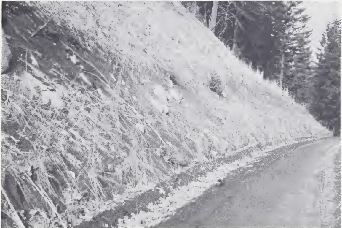
Photo 32.--Roadbank erosion control by vegetative methods on the Bear Creek road. FS Parkdale Ranger District photo. no. 3
