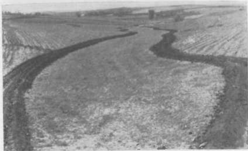
FIGURE 14.—This seeded drainageway is protected from run-off by temporary ditches along the sides of the seeded area. After the vegetation has become established the temporary ditches will be plowed in, and the run-off will then flow down the vegetated drainageway.
