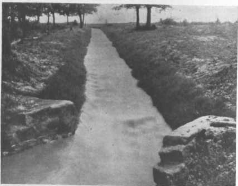
FIGURE 25.—This is the type of structure most commonly used if structural protection is necessary in farm drainageways.
