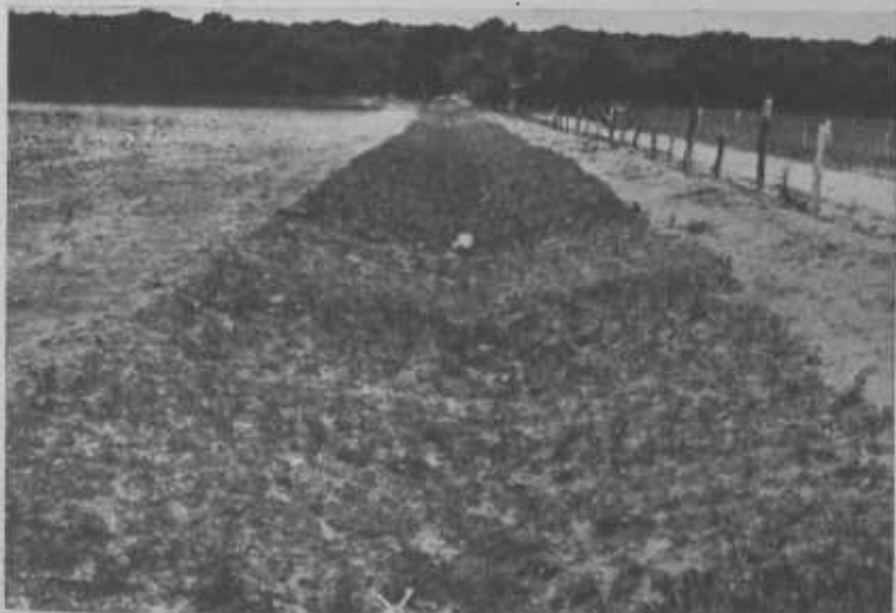
FIGURE 5.—V-shaped vegetated channels such as this are sometimes used where a satisfactory plant cover can be provided, where the run-off is small, and where it is desirable to concentrate the discharge on a restricted area.
