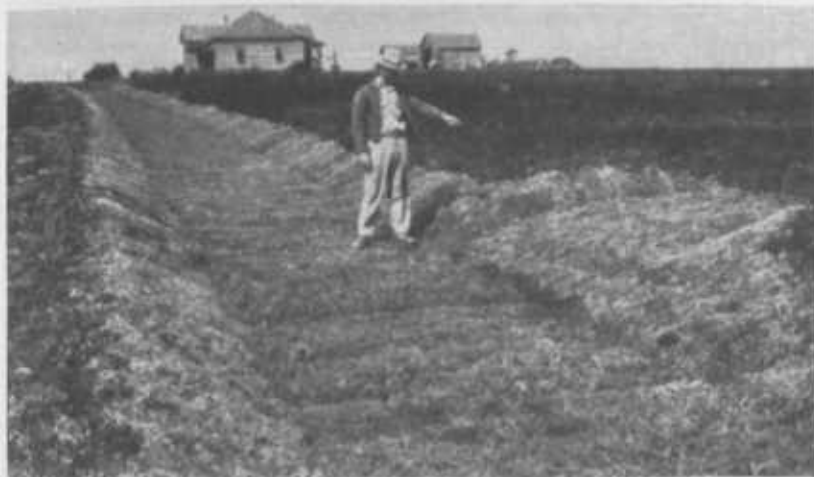
FIGURE 13.—A sodded terrace-outlet channel. Note how the terrace channel is shaped and protected at the discharge end. The broad, flat, sodded section spreads the run-off as it enters the outlet channel and prevents overfalls from advancing up the terrace channel.
