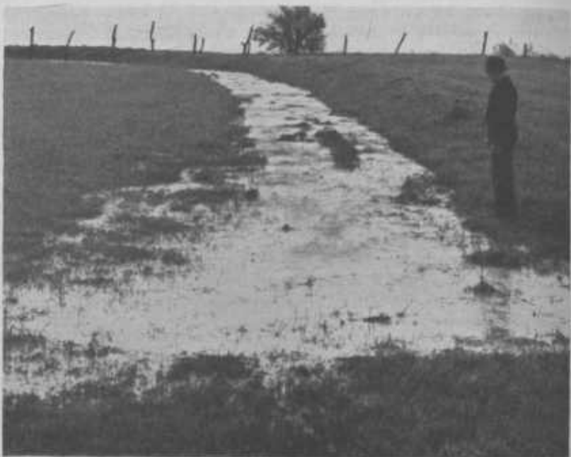
FIGURE 11.—Run-off is here discharging from an individual terrace over a well-sodded slope. The outlet end should be located and shaped so as to spread the discharge in as thin a sheet as possible over the slope.
