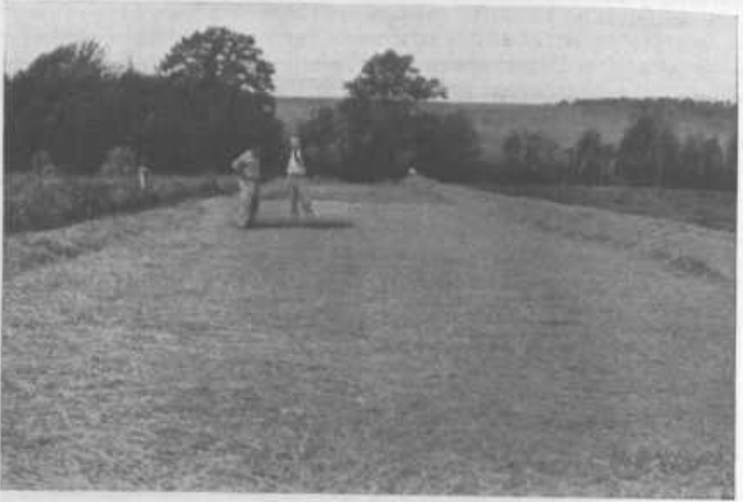
FIGURE 15.—A seeded drainageway protected by a straw mulch held in place by fine-mesh poultry wire. The wire will be removed when the vegetation becomes established.
