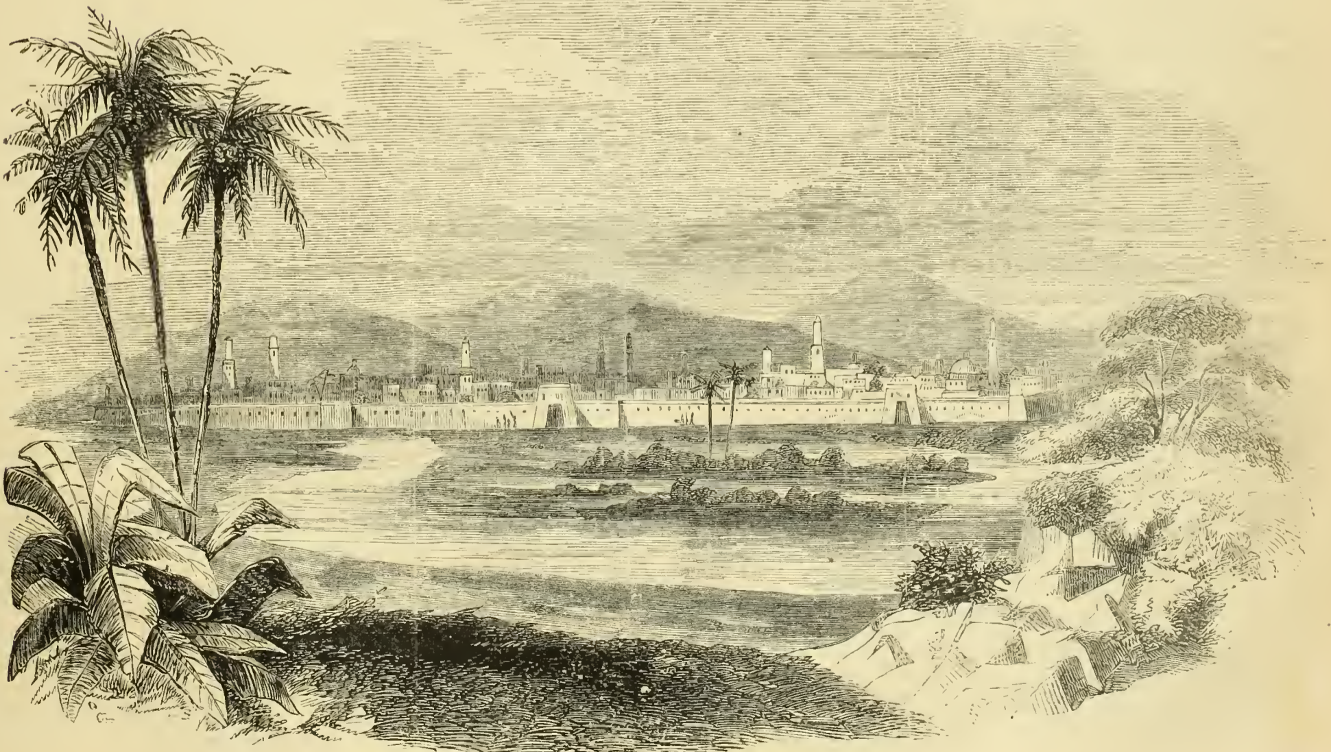
VIEW OF THE CITY OF KHAMTMANDU, THE CAPITAL OF NEPAUL.
