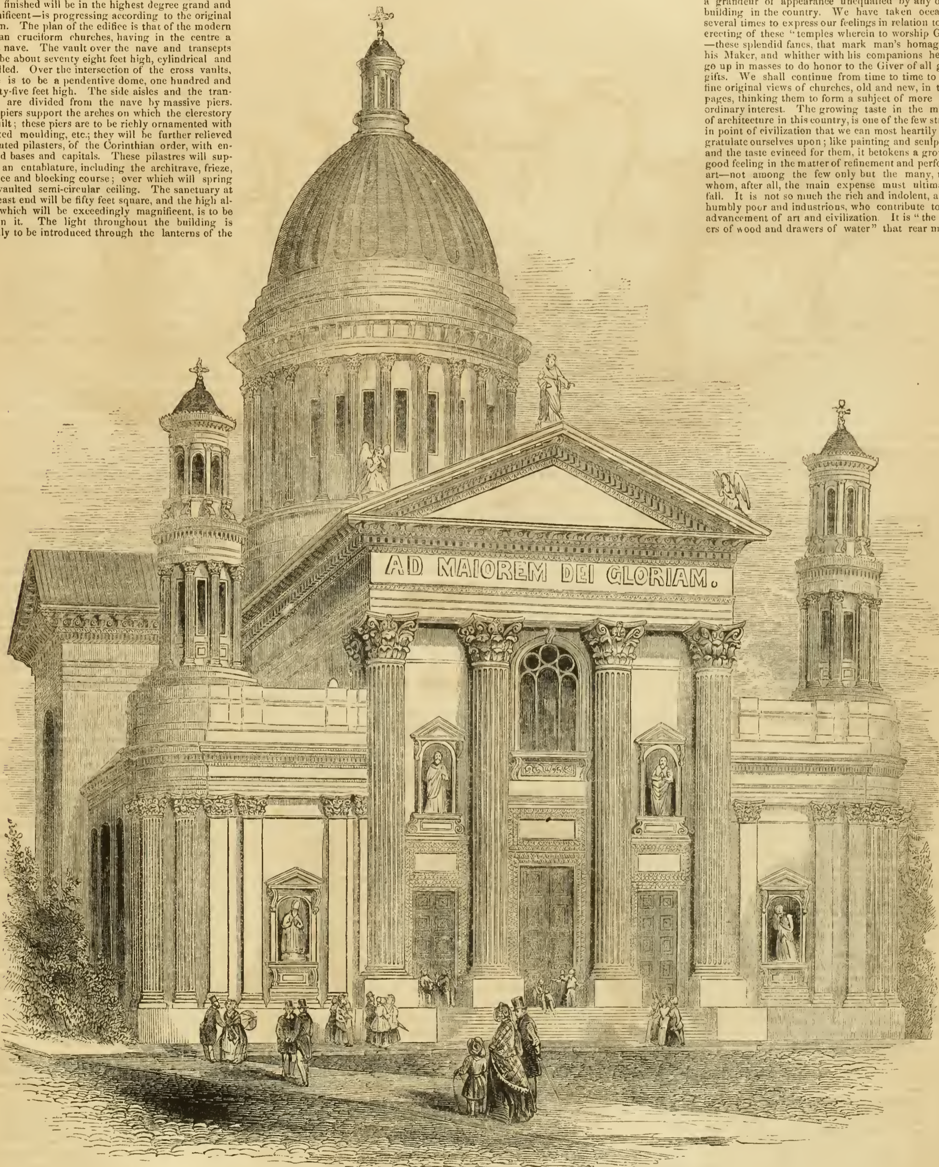
CATHEDRAL OF ST. PETER AND ST. PAUL, SCHUYLKILL, FIFTH, NEAR RACE STREET, PHILADELPHIA.
