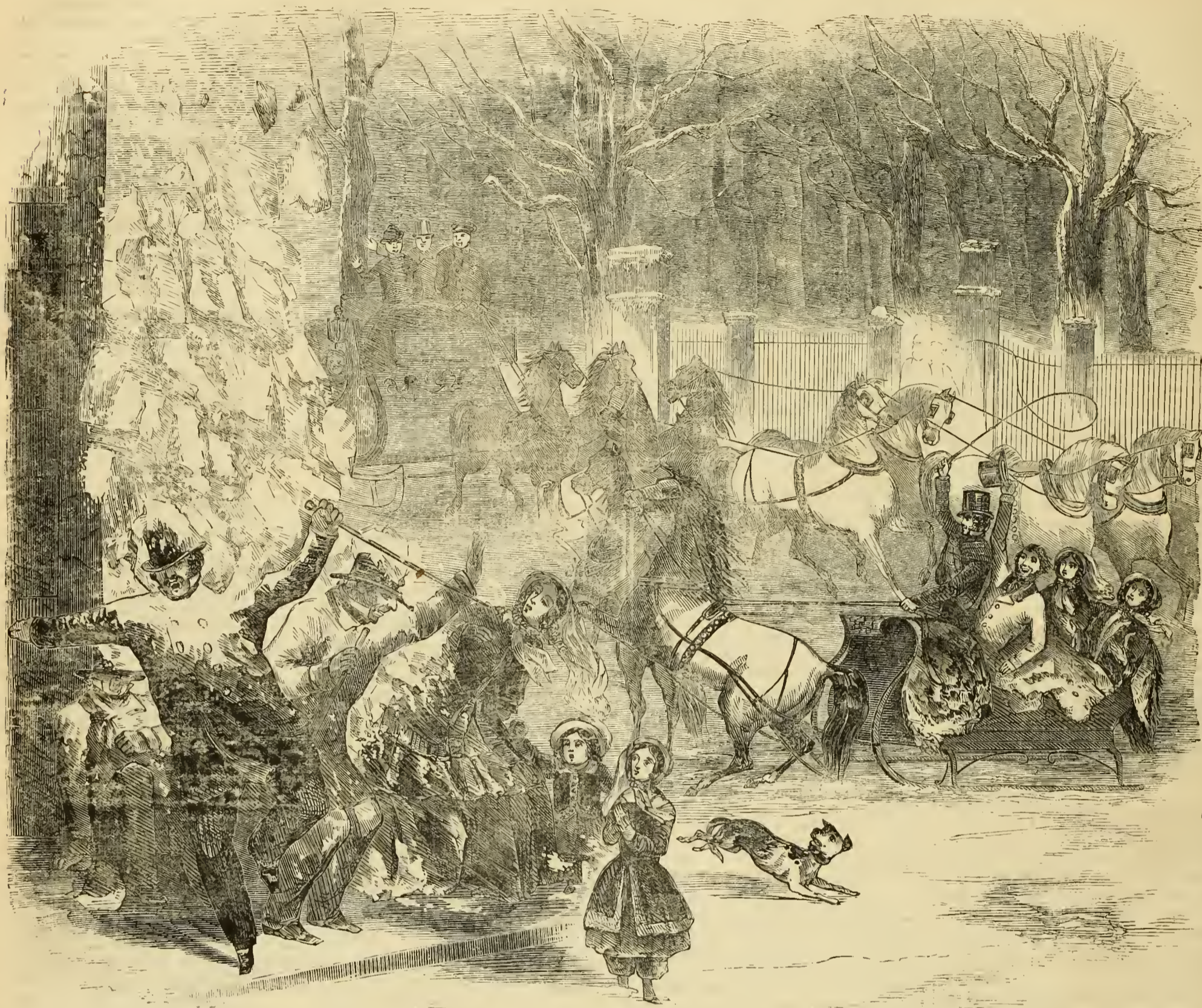
REPRESENTATION OF AN AVALANCHE OF SNOW FROM THE ROOF OF PARK STREET CHURCH.
