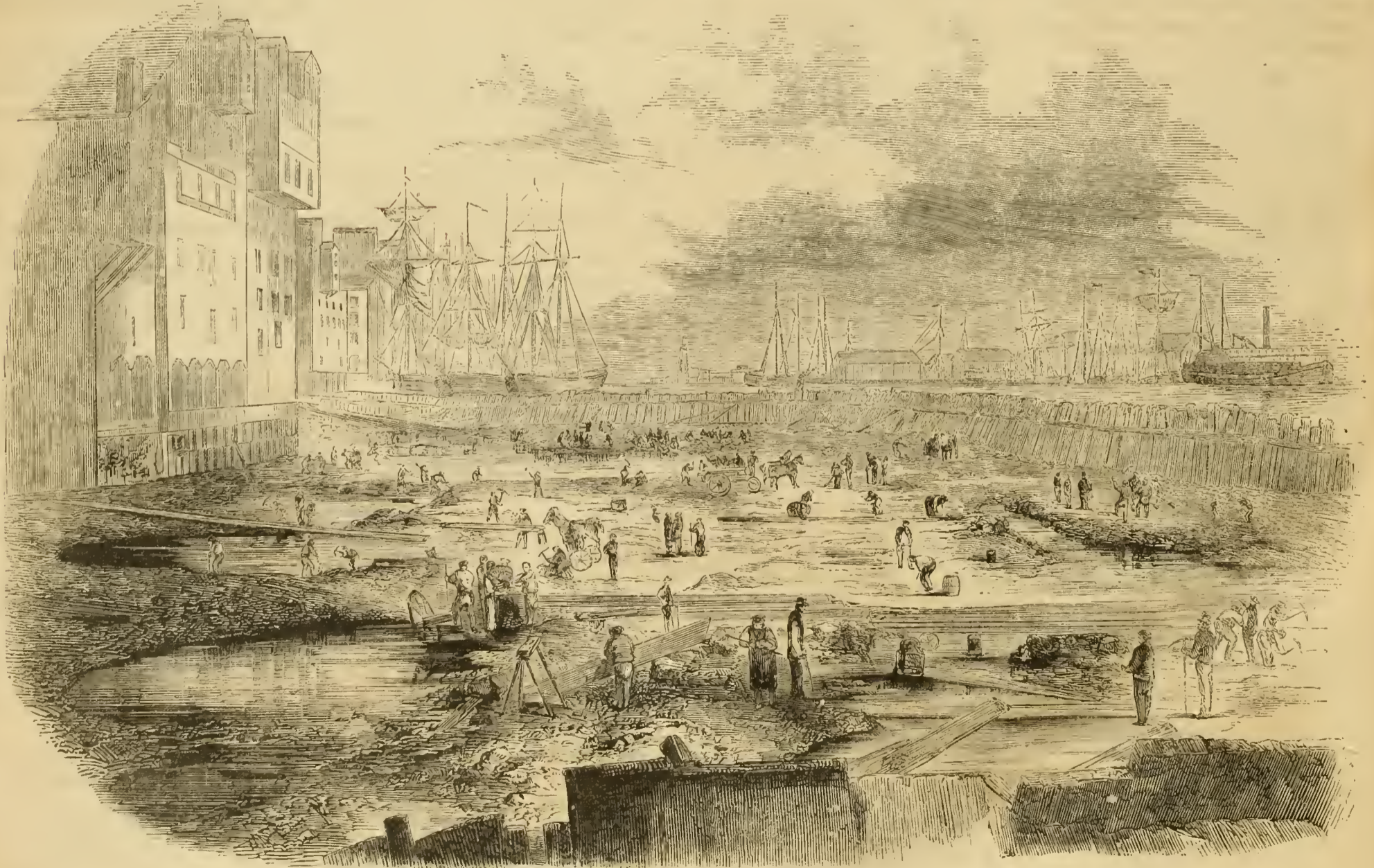
VIEW OF THE COFFER DAM, AT OSWEGO, N. Y.
