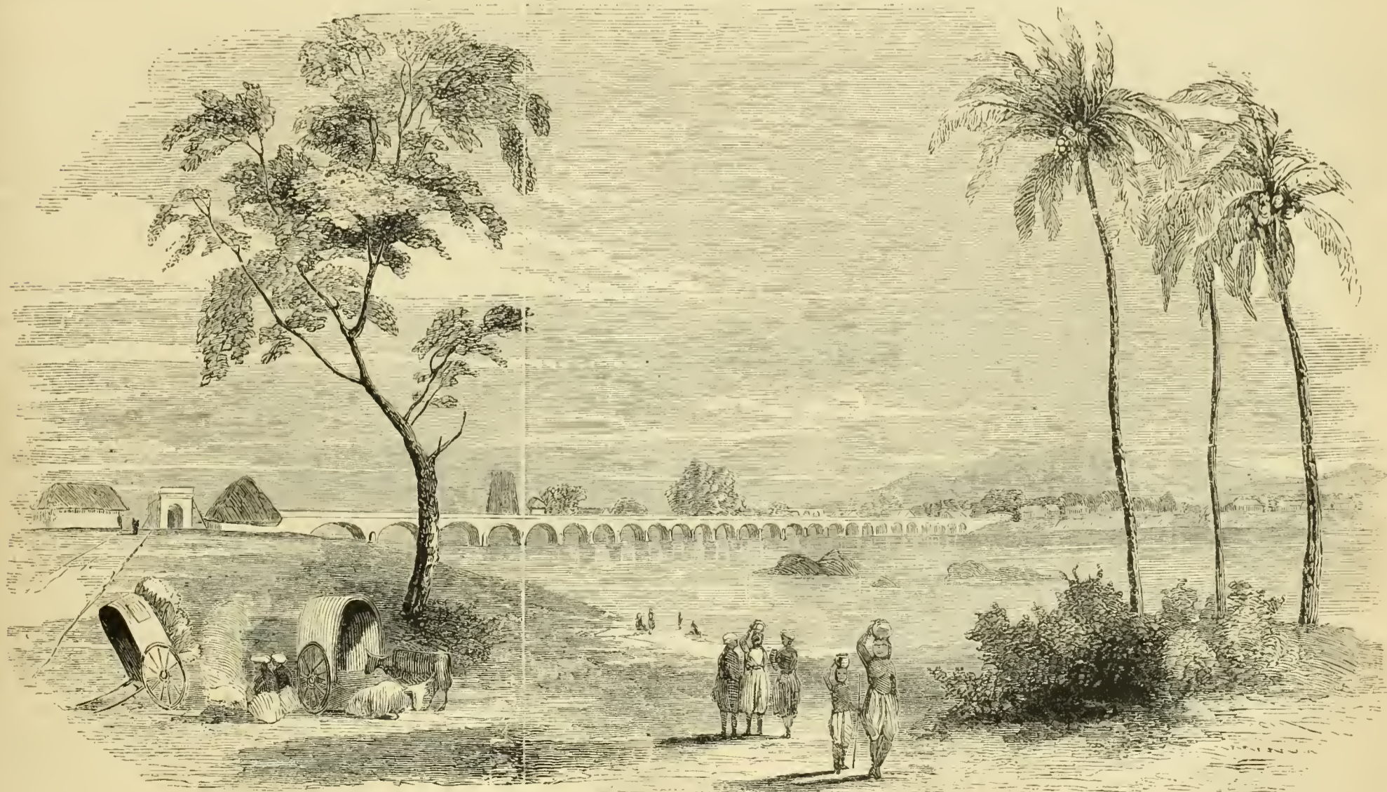
BRIDGE RECENTLY ERECTED OVER THE RIVER CORVERY, NEAR BHOWANEE, MADRAS
