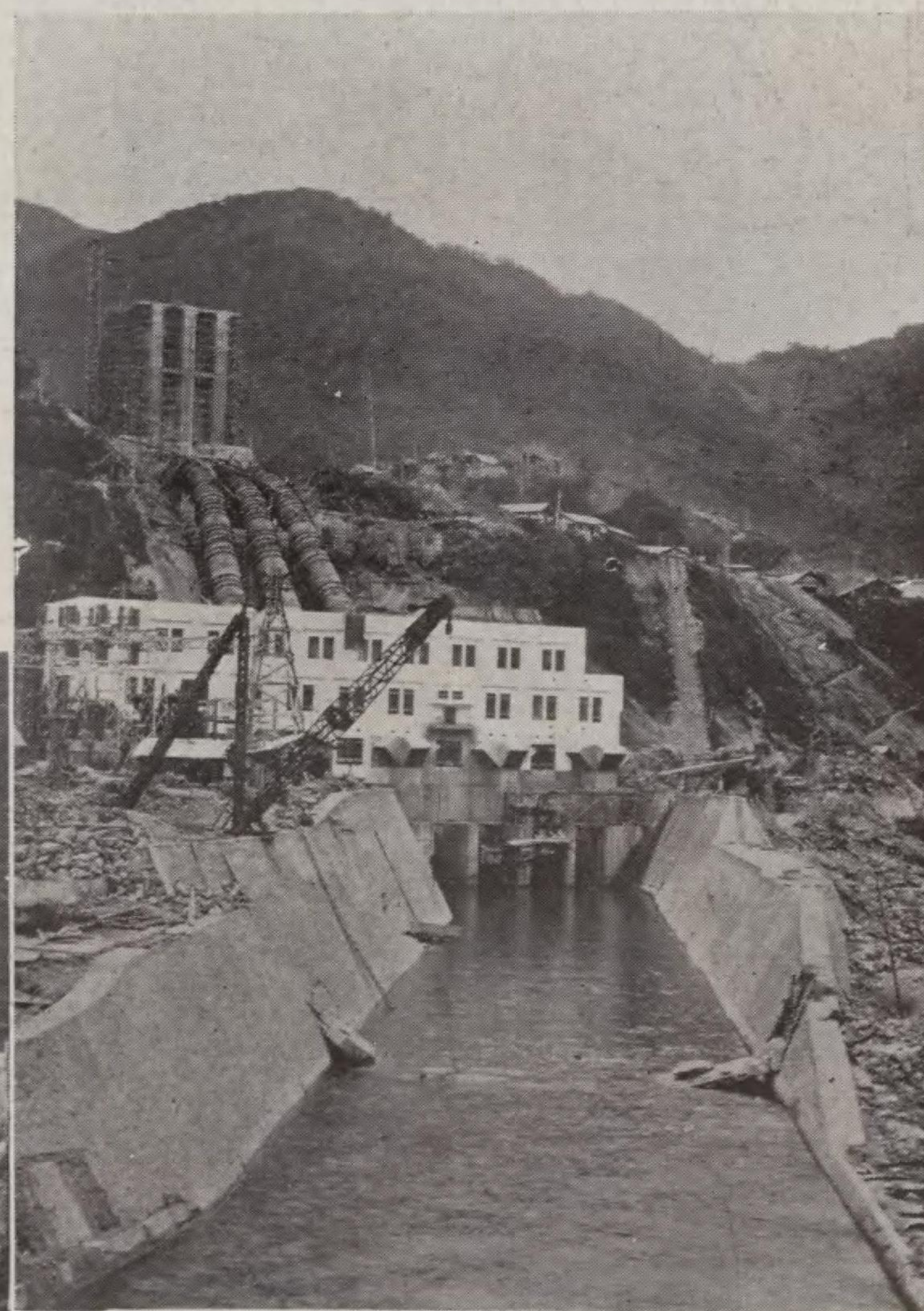
Front view of the Soyama Power Station. Total capacity: 60 000 kVA Effective head: 66.85 meters
