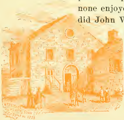
THE FIRST METHODIST CHURCH
