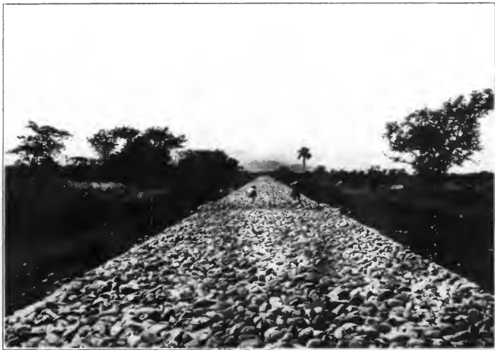
ONE OF THE NEW ROADS UNDER CONSTRUCTION IN CUBA.
