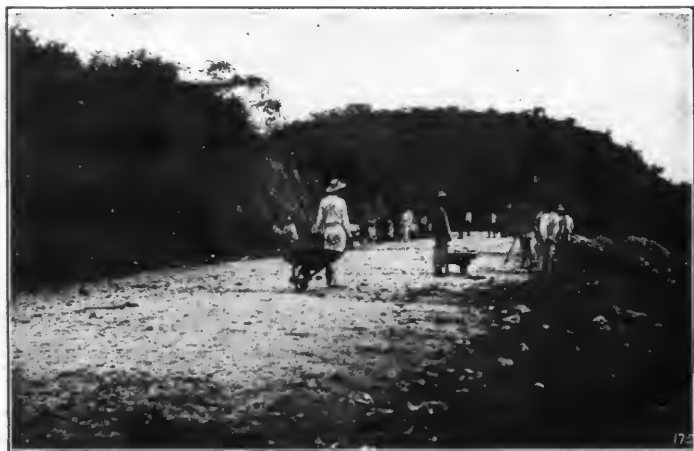
ROAD BUILDING IN HONDURAS.
