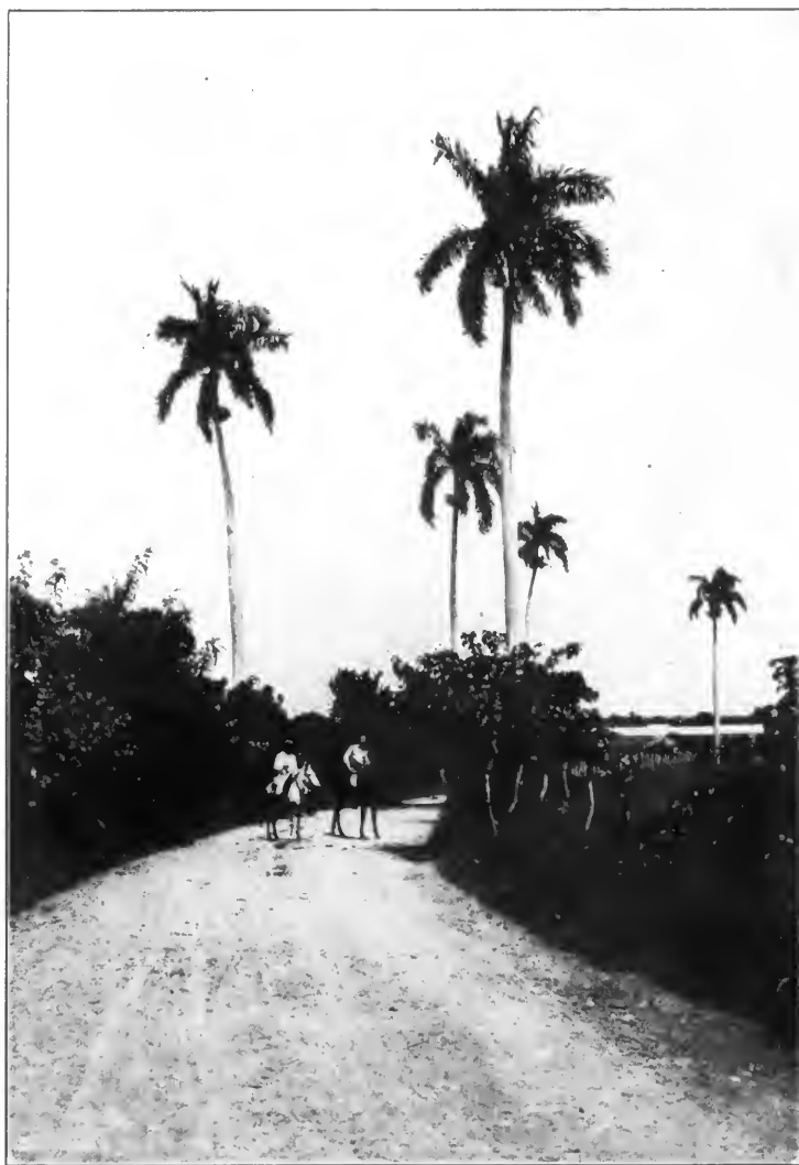
THE FINISHED ROADBED OF THE BAYAMO-MANZANILLO HIGHWAY.
