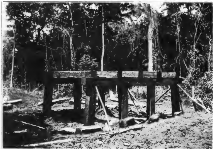
BUILDING CULVERT ON THE HIGHWAY FROM BAYAM TO MANZANILLO
