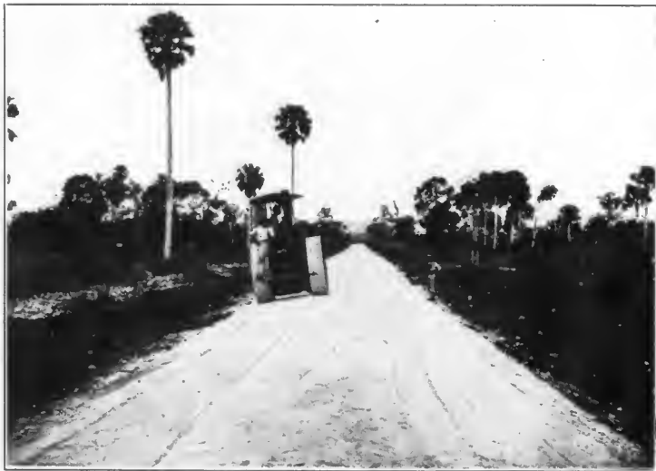
MODERN ROAD CONSTRUCTION IN CUBA.
