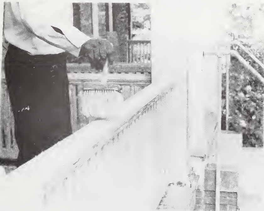
Figure 6. Application of paint remover on painted wood railing by brush.
