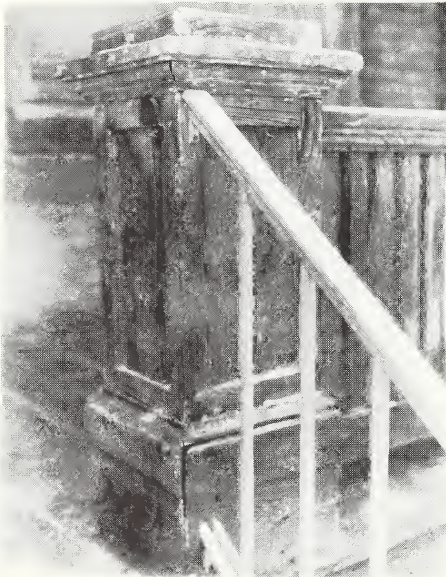
Figure 11. Porch rails after application of three coats of paint remover and water spray flush. Hand scraping was necessary to completely remove paint from the base of railings.
