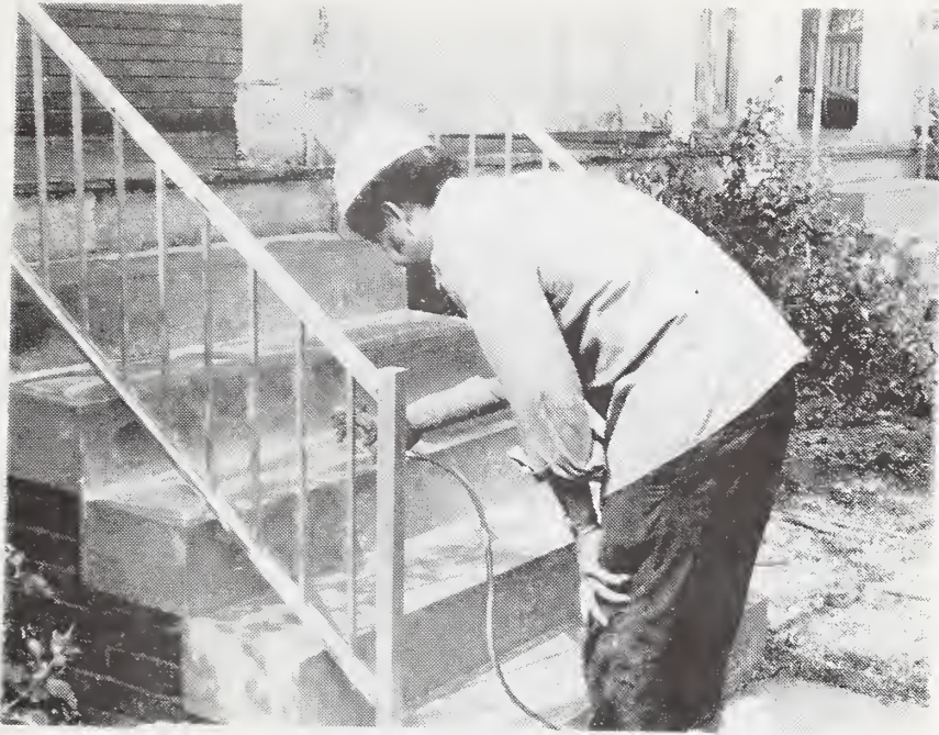
Figure 5. Application of paint remover on painted concrete stairs with spray equipment.
