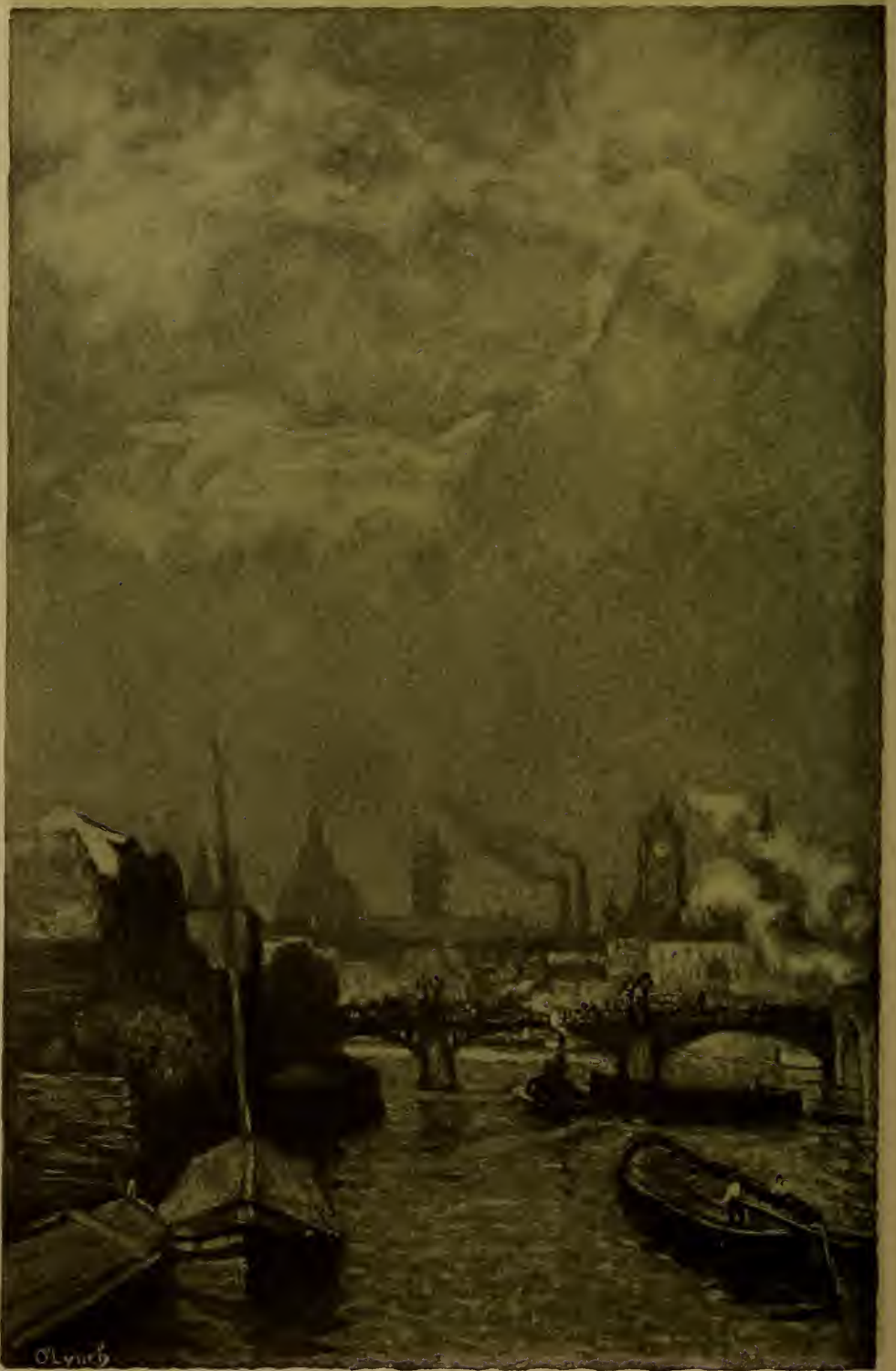
THE JANOWITZ BRIDGE OVER THE SPREE
