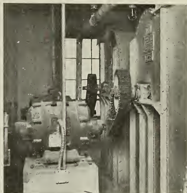
MORSE DRIVES ON ELEVATOR HEADS
