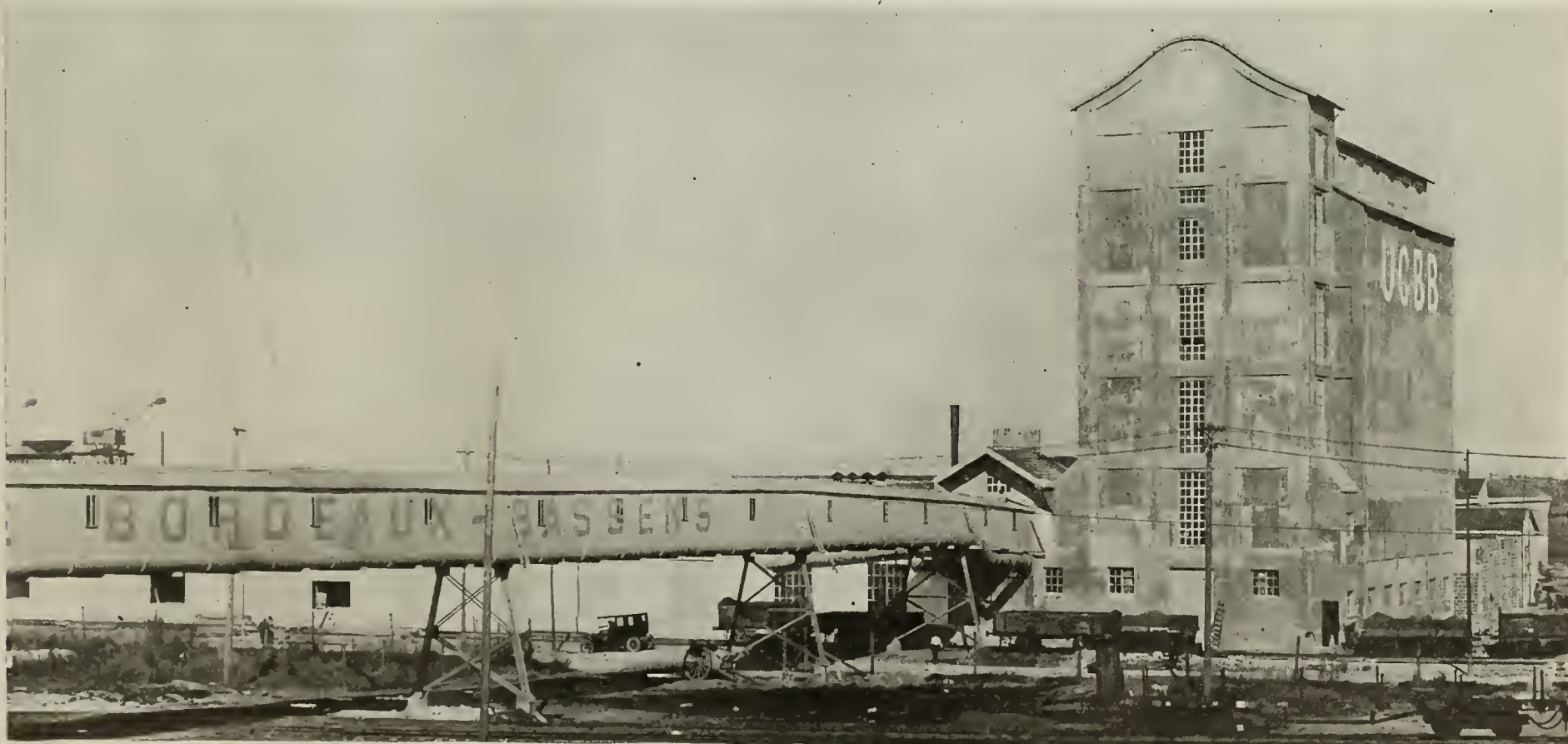
VIEW OF ELEVATOR AT BORDEAUX, FRANCE, WITH CONVEYOR GALLERY LEADING TO DOCK
