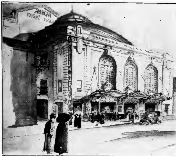
William Morris house now in course of construction on Ellis street, scheduled to be opened in July.
