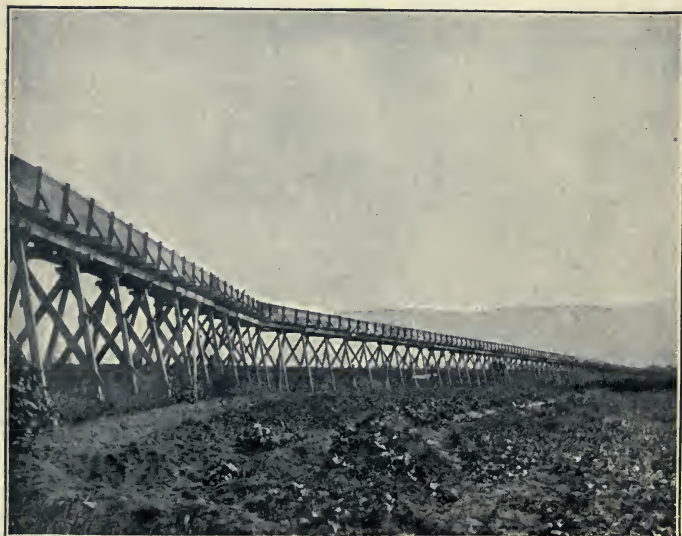
IRRIGATION FLUME, FORT ROMIE.
