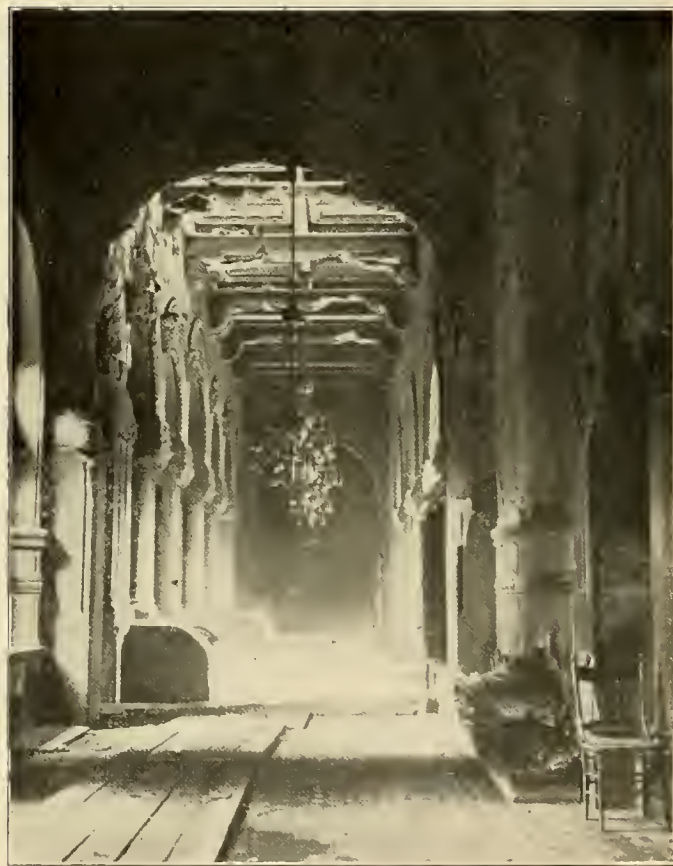
Great western staircase, corridor fourth floor, after cleaning up
