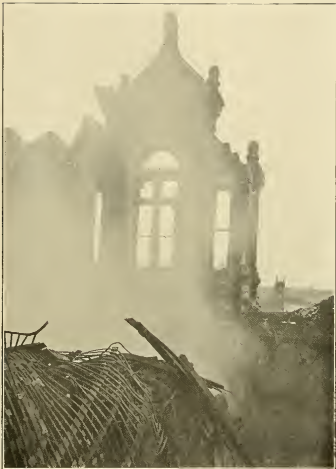
Southwest dormer window looking south. The roof had fallen
