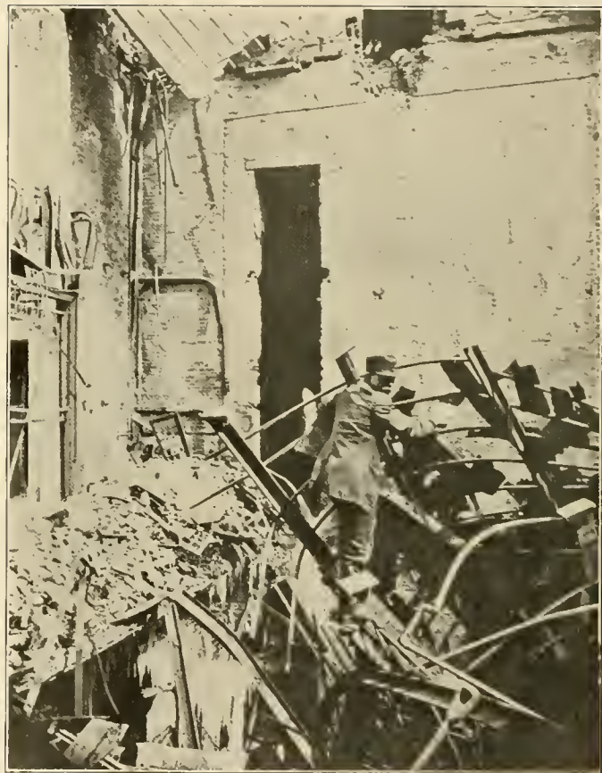
The remains of the Department of State Board of Regents, 4th floor
