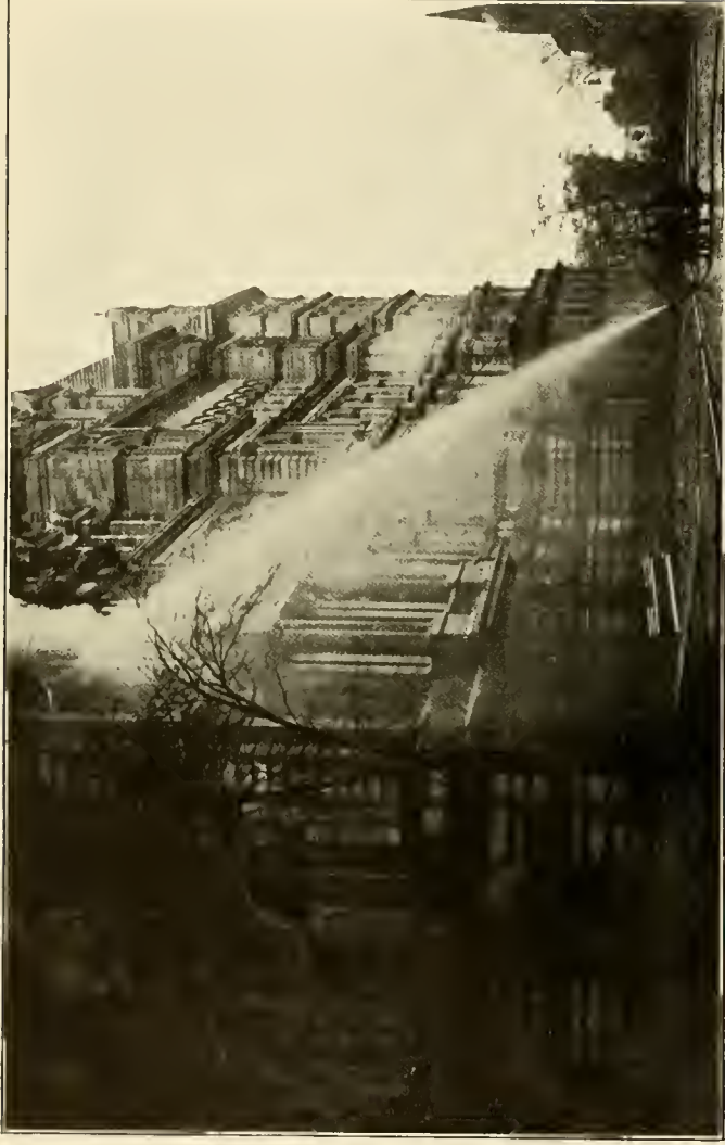
Firemen fighting the fire in the northwest corner of the Capitol
