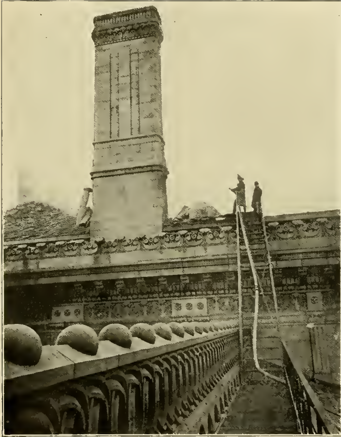
Firemen at work on southwest tower
