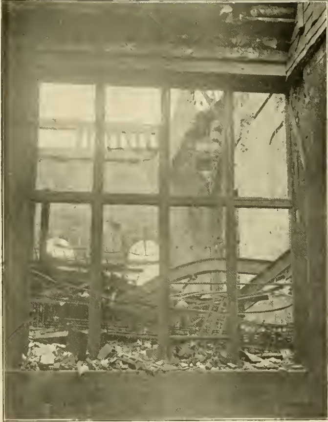
Looking through window in library
