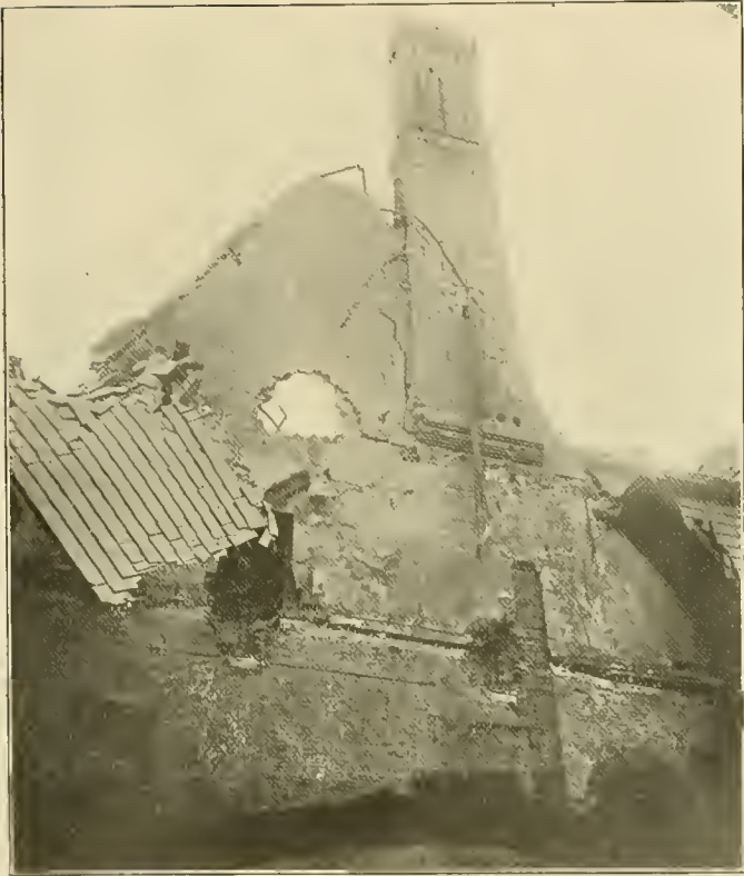
The fallen roof of southwestern part of Capitol
