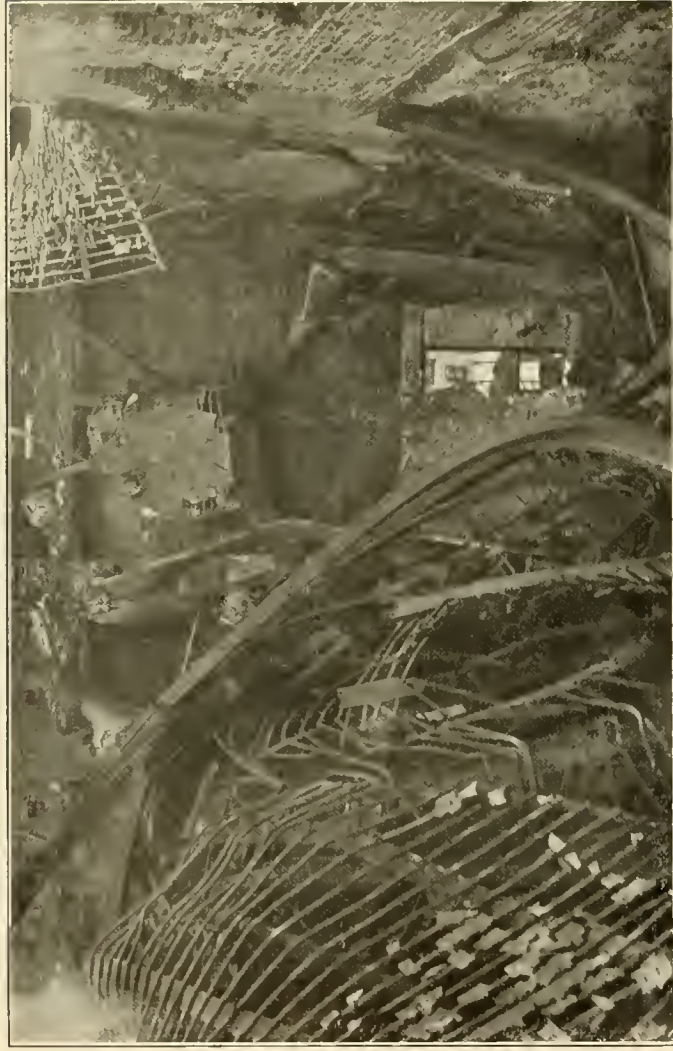
Twisted iron in the southwest tower
