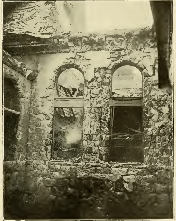
Showing effect of fire on the stone
