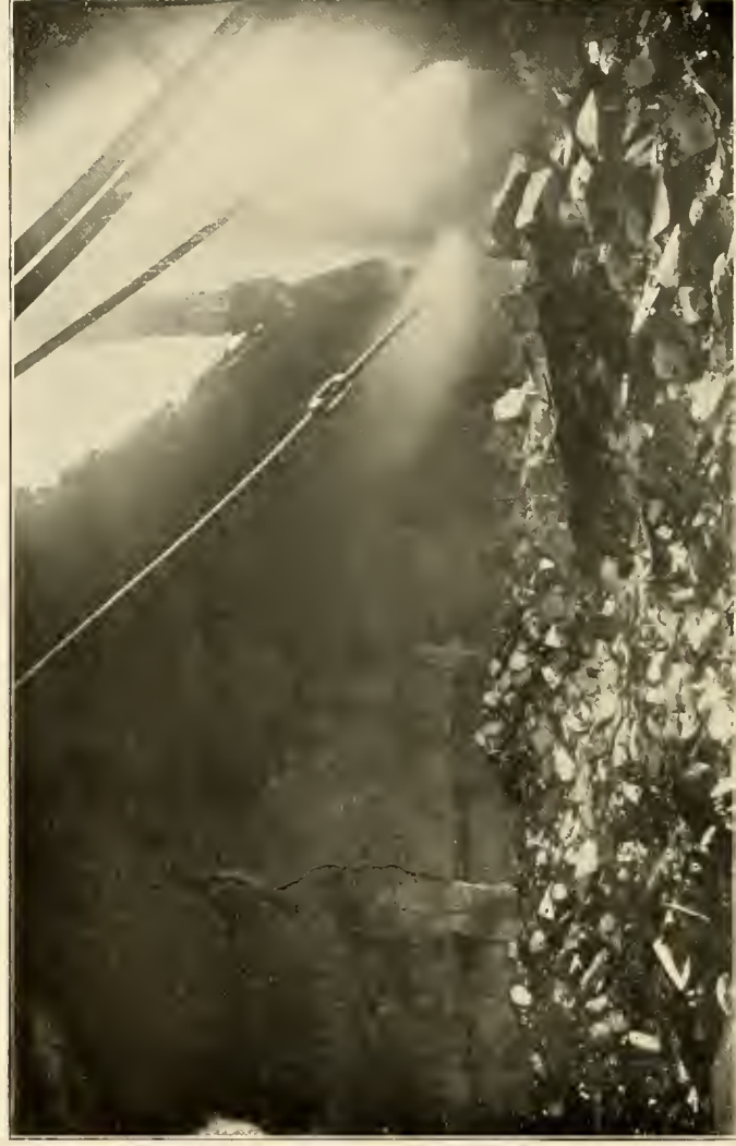
Showing damage fire can do
