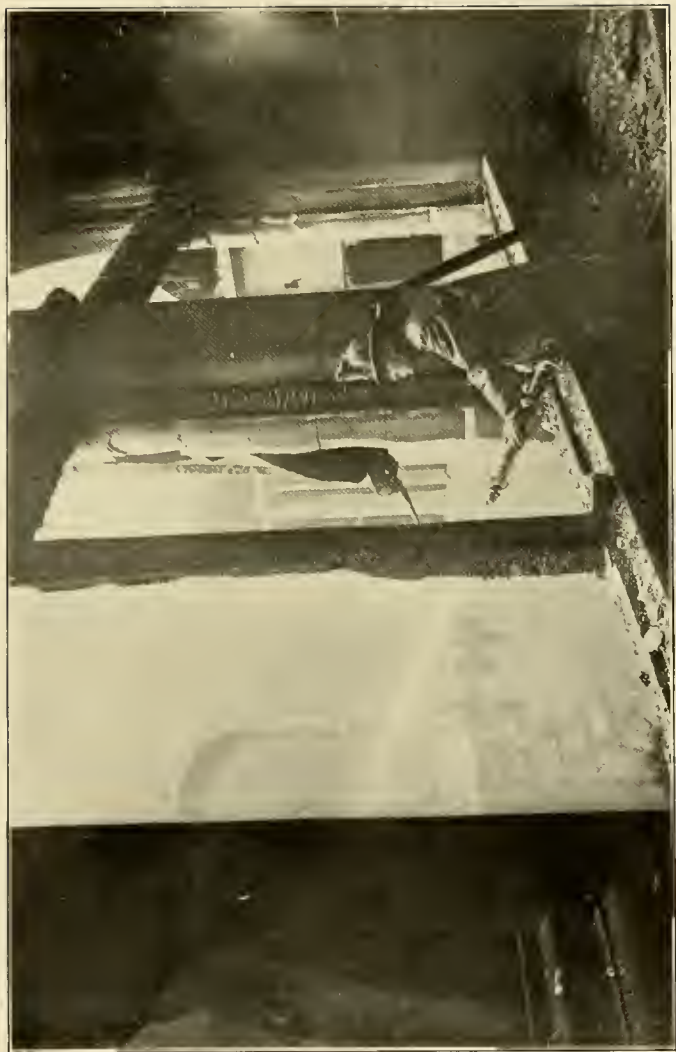
Fireman at work cooling down the ruins, playing stream through air shaft on third floor of Great Western Staircase
