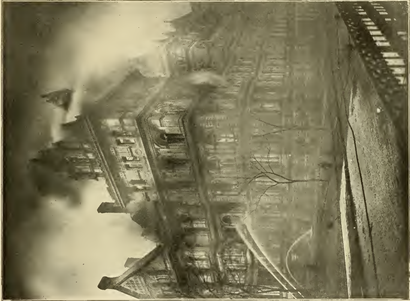
Just as the roof of the southwest tower fell in
