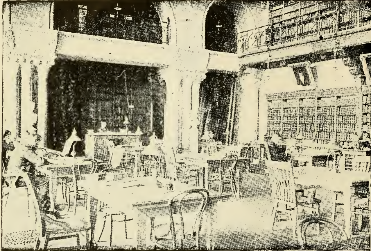
Library reading room before the fire
