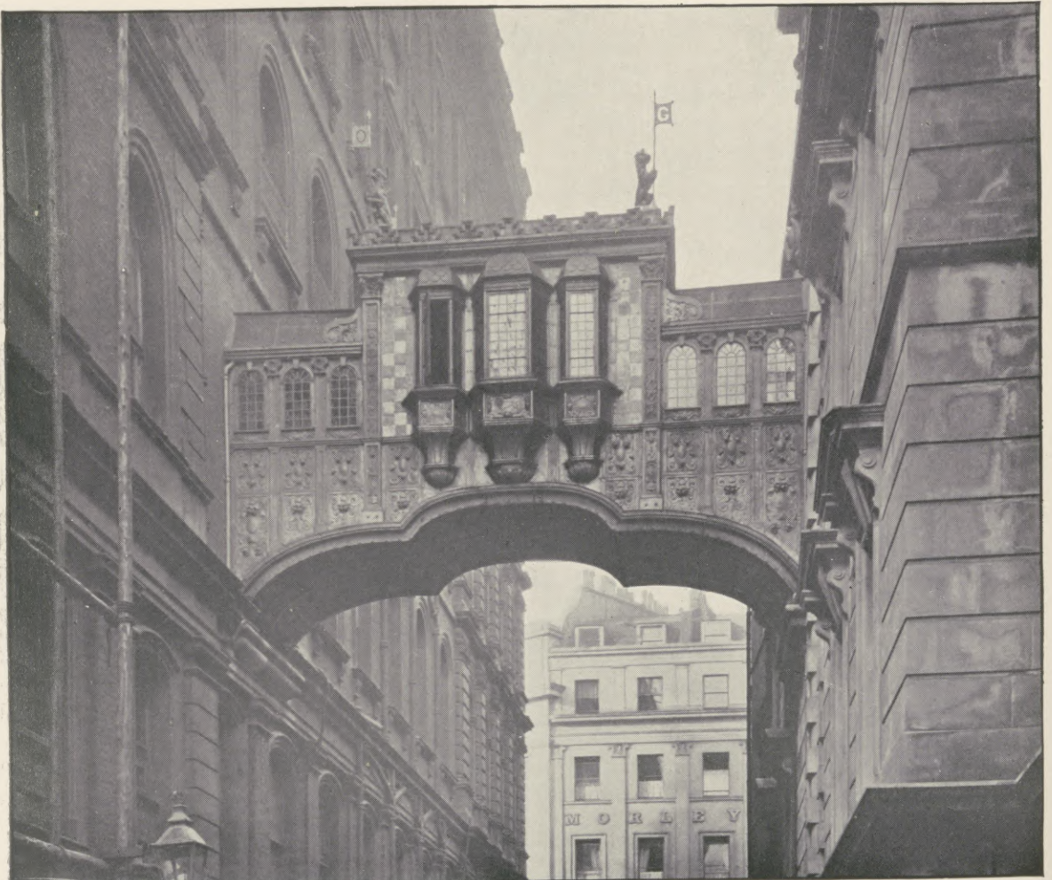
COVERED BRIDGE OF IRON, SHEATHED IN CAST LEAD, GRAND HOTEL, LONDON. Designed by WILLIAM WOODWARD, and executed by STARKIE GARDNER AND Co.
