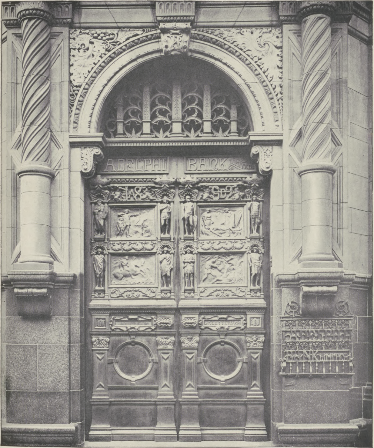
CAST BRONZE GATES, ADELPHI BANK, LIVERPOOL. Designed by W. D. CARÖE, the figures by STIRLING LEE, executed by STARRIE GARDNER AND Co.
