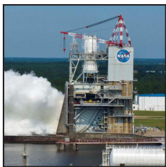
J-2X Test Stennis Space Center April 2013
