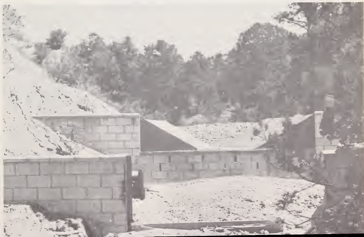
Figure 8.--A view looking upstream into the sediment basin after at least 18 tons of sediment had passed through the flume in a single flow. (The downstream sediment basin wall failed.) Flume sidewalls were scratched, but there were no dimensional changes.
