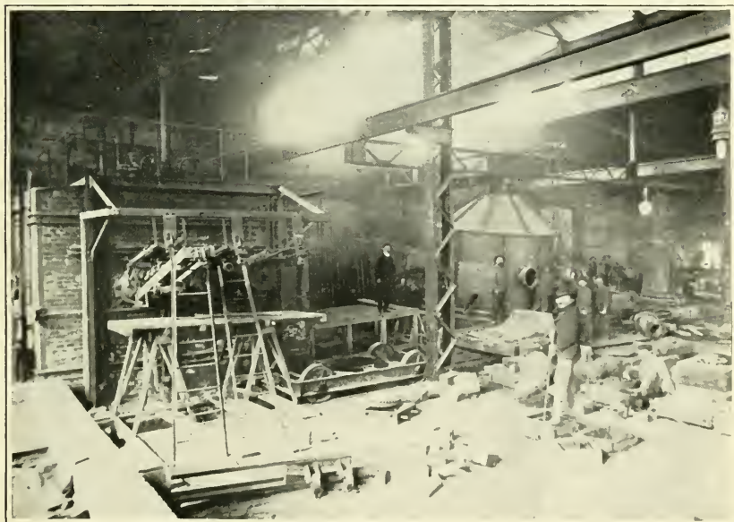
STASSANO 1,000-HORSEPOWER ELECTRIC FURNACE, FIXED TYPE.
