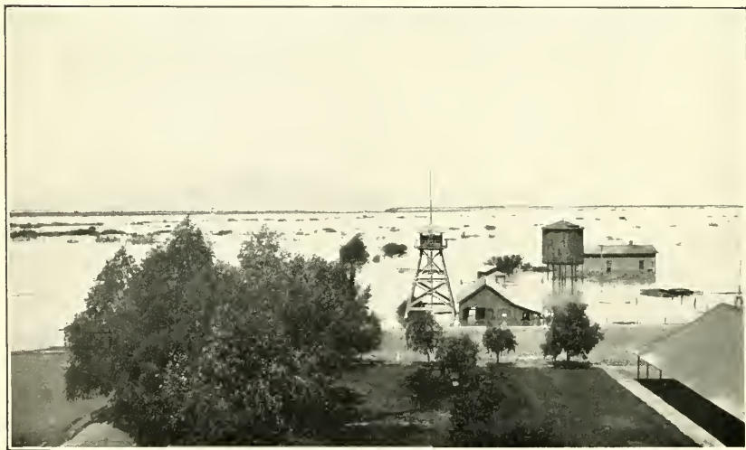
LOOKING SOUTHERLY OVER TEMPORARY DIKES IN THE SUBMERGED TOWNS OF CALEXICO AND MEXICALA.
