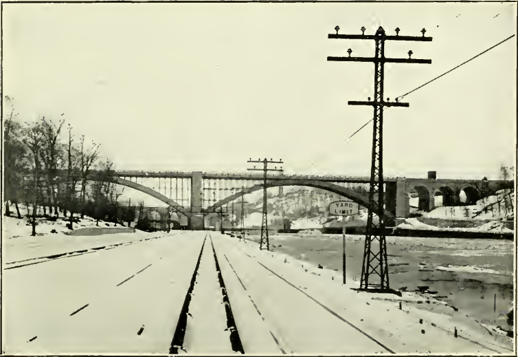
PROTECTED THIRD RAIL BURIED IN SNOW.
