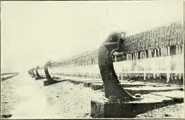
PROTECTED THIRD RAIL AFTER SLEET STORM.
