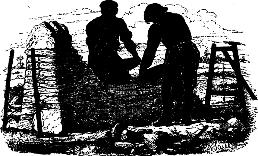
THE BUILDING A DRY-STONE DYKE.
