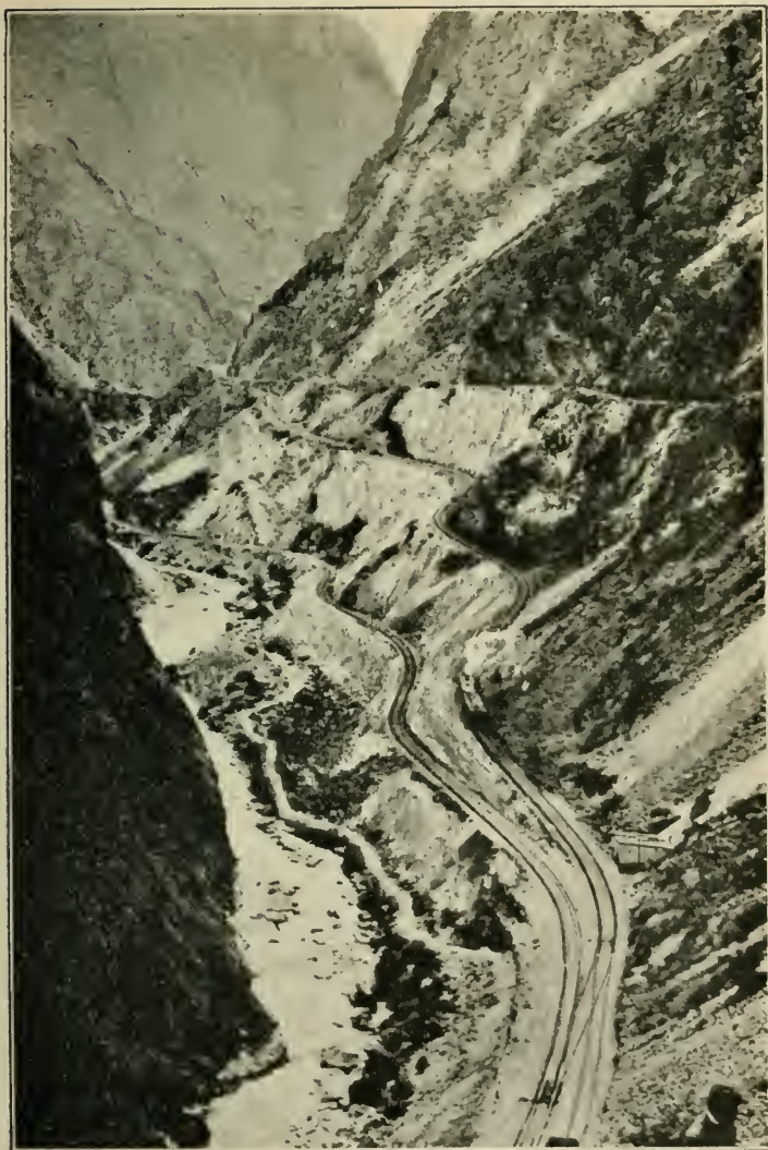
A railway in the Andes built by American engineers. The track zigzags back and forth to reach higher grades.
