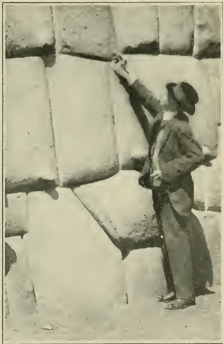
The Incas built walls of enormous stones without mortar, but so nicely fitted that the author cannot thrust a needle between them.
