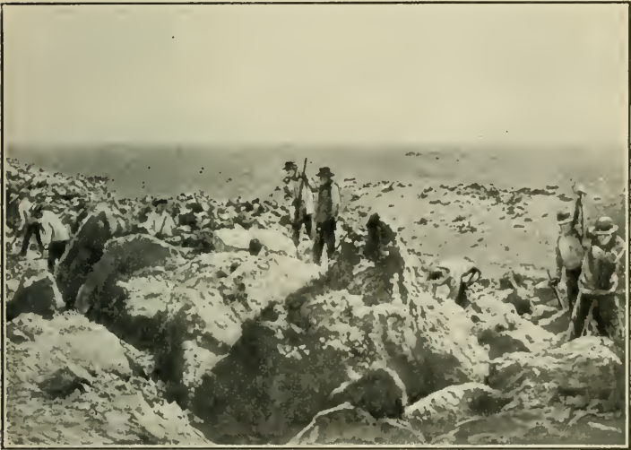
Opening up a trench in the nitrate beds after blasting.
