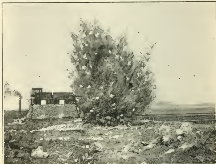
Blasting the nitrate rock.
