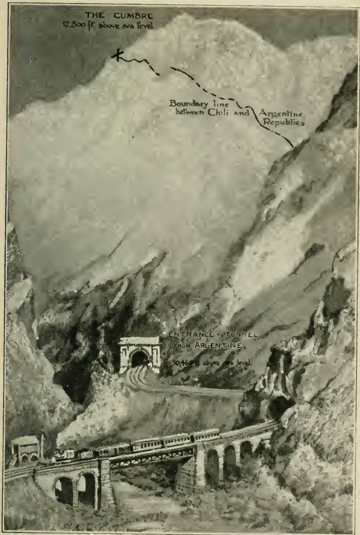
On the Transandine railway. The cross marks the site of the Christ of the Andes, 2000 feet above the tunnel.
