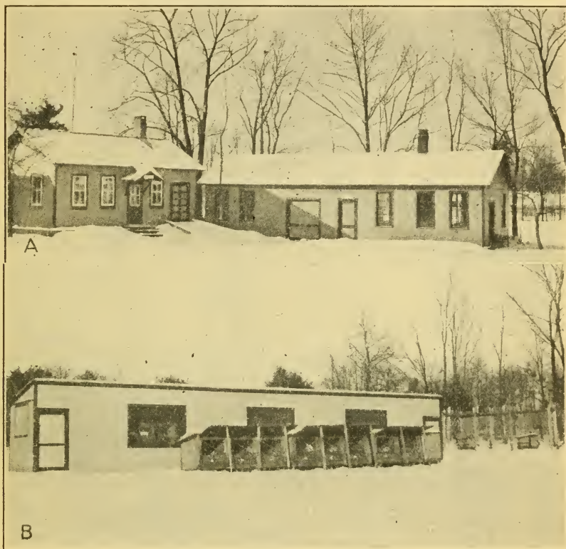
FIG. 2.—Structures on the experimental fur farm: A, Office and laboratory (at left) and building (at right) containing feed room, storerooms, and carpenter shop; B, rabbit building, for breeding does, with hutches for bucks in the foreground. The main ranch is seen at the extreme right (fig. 3)
