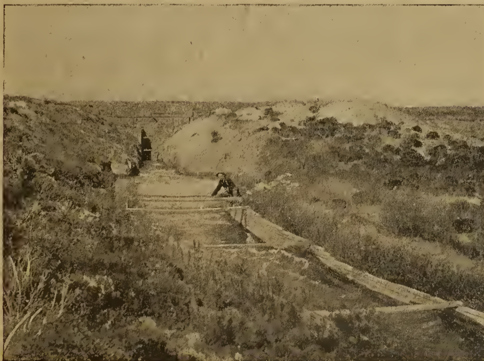
DISCHARGE-WAY AND MEASURING-WEIR
