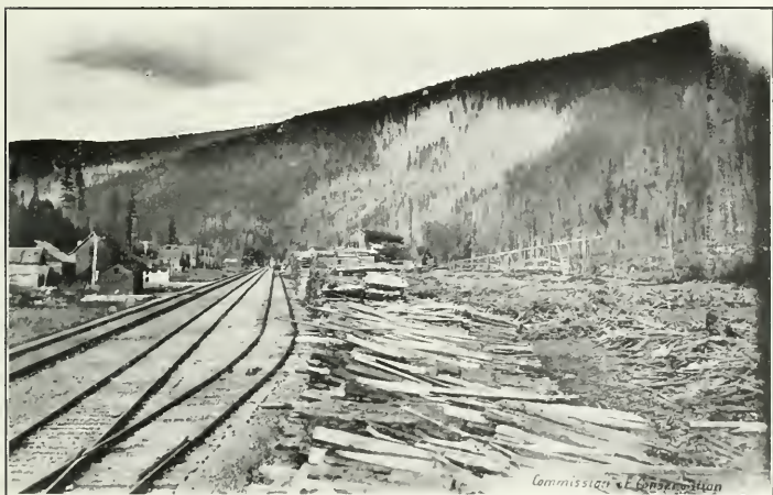
FIRE DANGER AND DAMAGE ADJACENT TO SAWMILL AND RAILWAY LINE Note burned slopes and large accumulation of inflammable sawmill debris.
