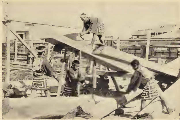
CARPENTERS AT WORK.
