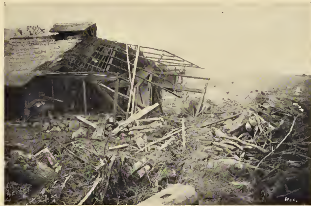
WRECKED BY AN EARTHQUAKE.
