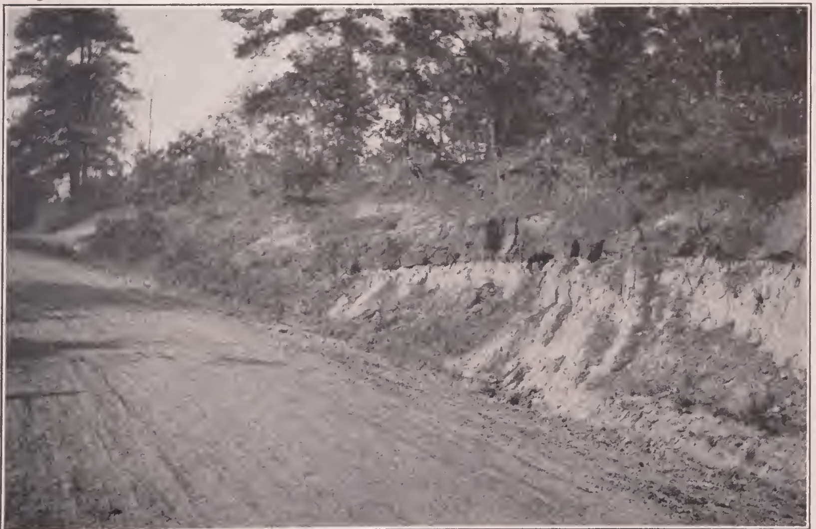
B. EXPOSURE IN CUT OF COLUMBUS-SEALE ROAD, FOUR MILES SOUTHWEST OF COLUMBUS, GA., IN RUSSELL COUNTY, ALA., SHOWING CONTACT BETWEEN LOWER CRETACEOUS BED AND THE OVERLYING EUTAW FORMATION.
