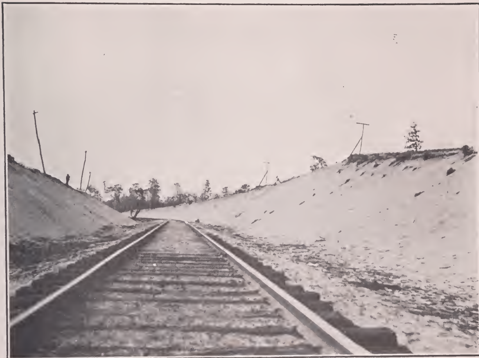
A. CUT OF MACON, DUBLIN & SAVANNAH RAILROAD THROUGH A SAND HILL ON EAST SIDE OF OCONEE RIVER, NEAR DUBLIN, LAURENS COUNTY.
