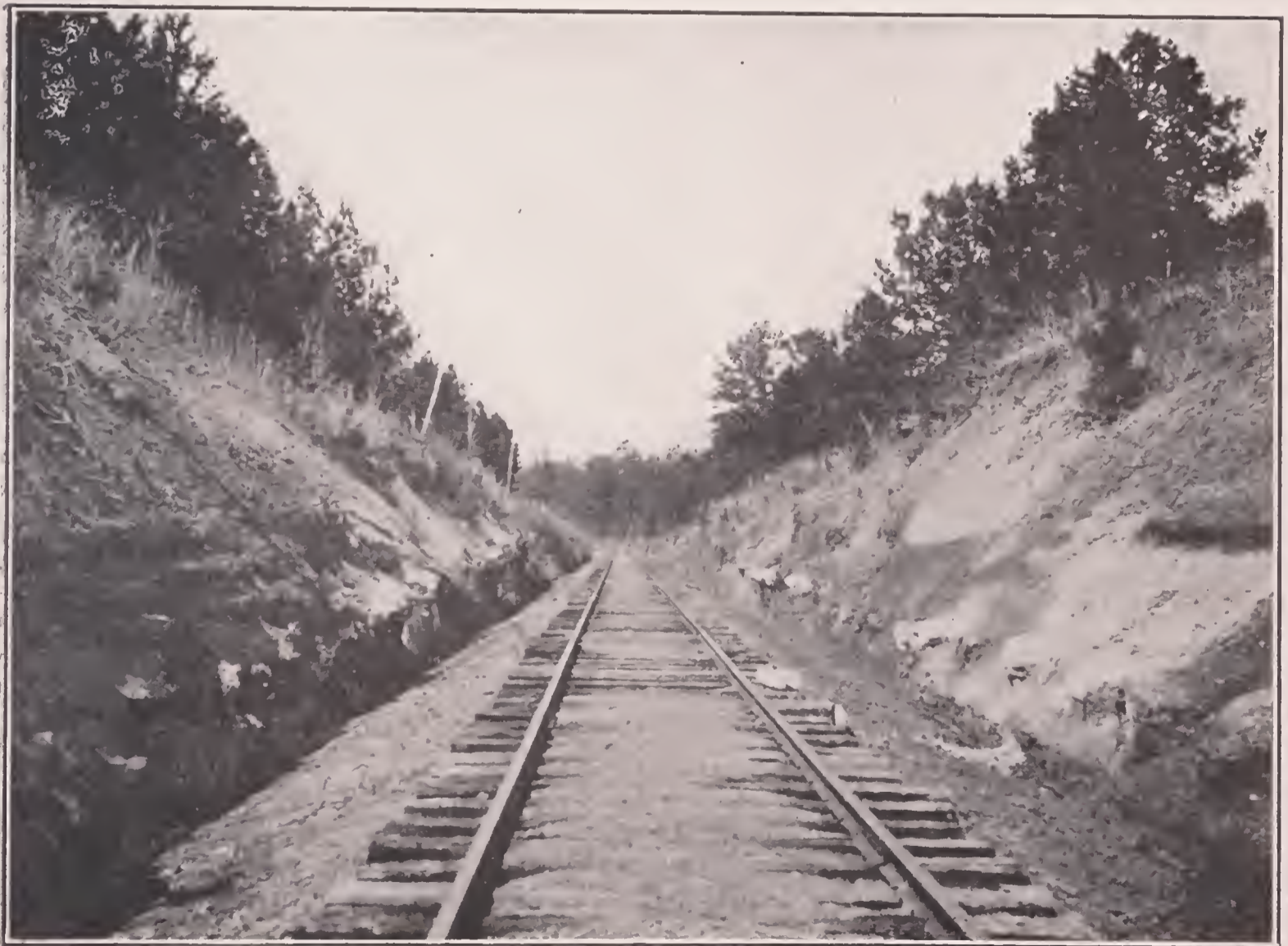
B. EXPOSURE IN CUT OF SEABOARD AIR LINE RAILWAY, TWO AND ONE-HALF MILES NORTHWEST OF CUSSETA, CHATTAHOOCHEE COUNTY, GA., SHOWING GRAY, MARINE SANDS WITH A LAYER OF CALCAREOUS CONCRETIONS NEAR THE BASE, BELONGING TO THE TOMBIGBEE SAND MEMBER OF THE EUTAW FORMATION.
