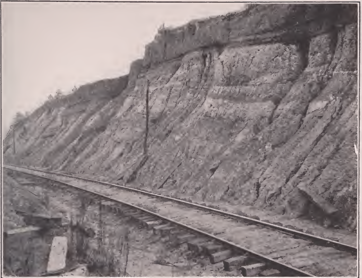
A. CUT OF SEABOARD AIR LINE RAILWAY AT MANTA STATION, CHATTAHOOCHEE COUNTY. STRATA OF THE CUSSETA SAND MEMBER OVERLAIN BY MARINE MATERIALS OF THE RIPLEY FORMATION.
