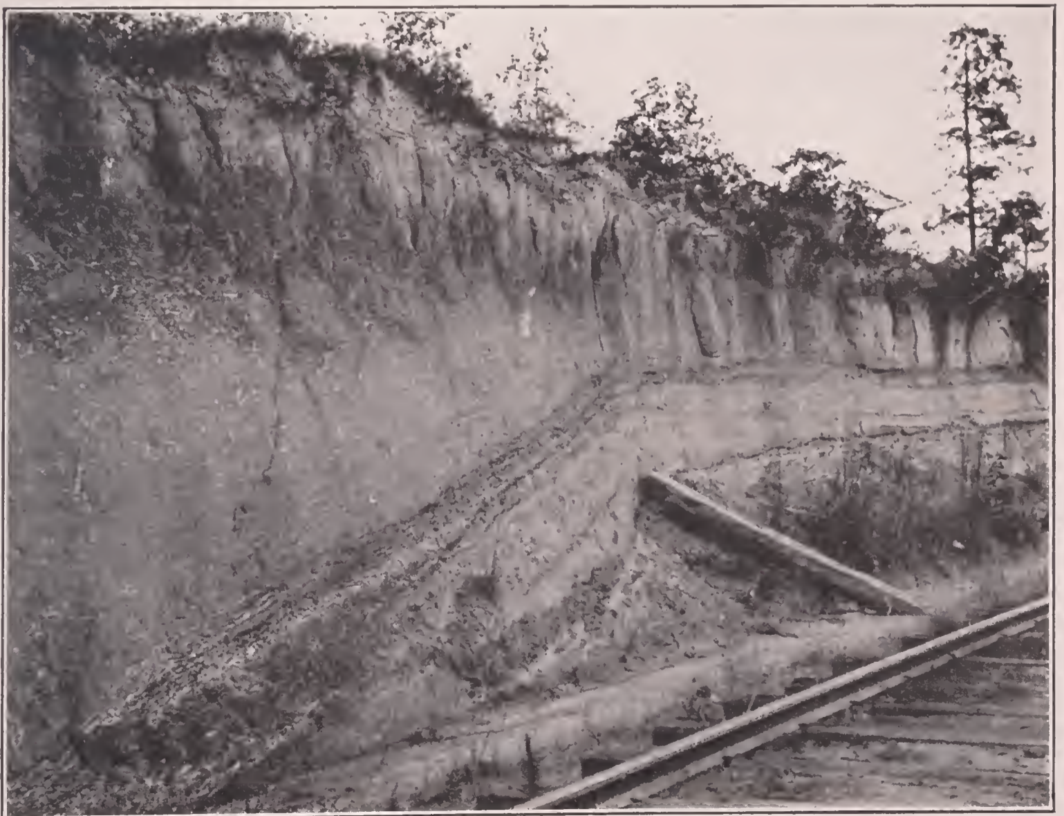
B. CUT ON SEABOARD AIR LINE RAILWAY, THREE MILES EAST OF CUSSETA, SHOWING WEATHERED SAND AND LAMINATED CLAY BEDS OF THE CUSSETA SAND MEMBER OF THE RIPLEY FORMATION.
