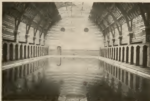
Fig. 2. Men's Swimming Bath, Leeds, England. (Lighted by sky-light only.) By courtesy of "Modern Sanitation."
