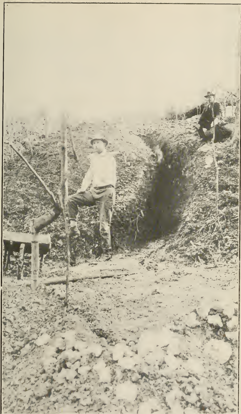
Fig. 3. Tunnel of Hall and Timberlake kaolin mine in Section 27, VanBuren Township. White masses in front are fragments of kaolin taken from mine.
