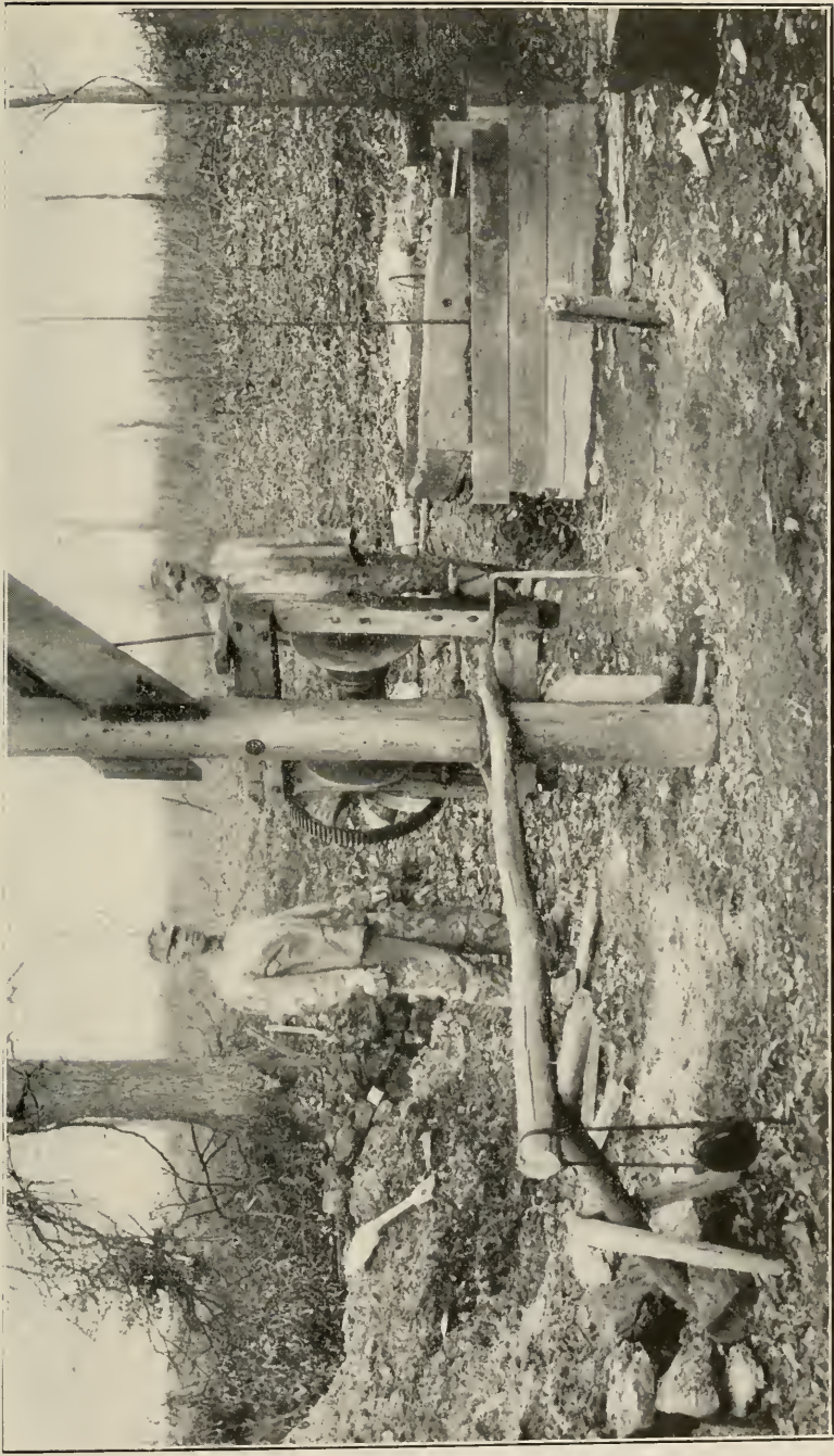
Fig. 2. Coal mine on the David Koonz Farm. Property of Hall and Timberlake. Shaft seventeen feet deep. Coal at rear of man on left hand.
