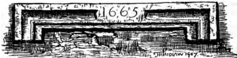
DOOR LINTEL, OLD HARWOOD HOUSE
