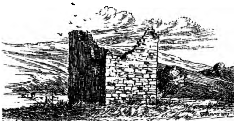
Fulton Tower. Bedrule. 1907.
