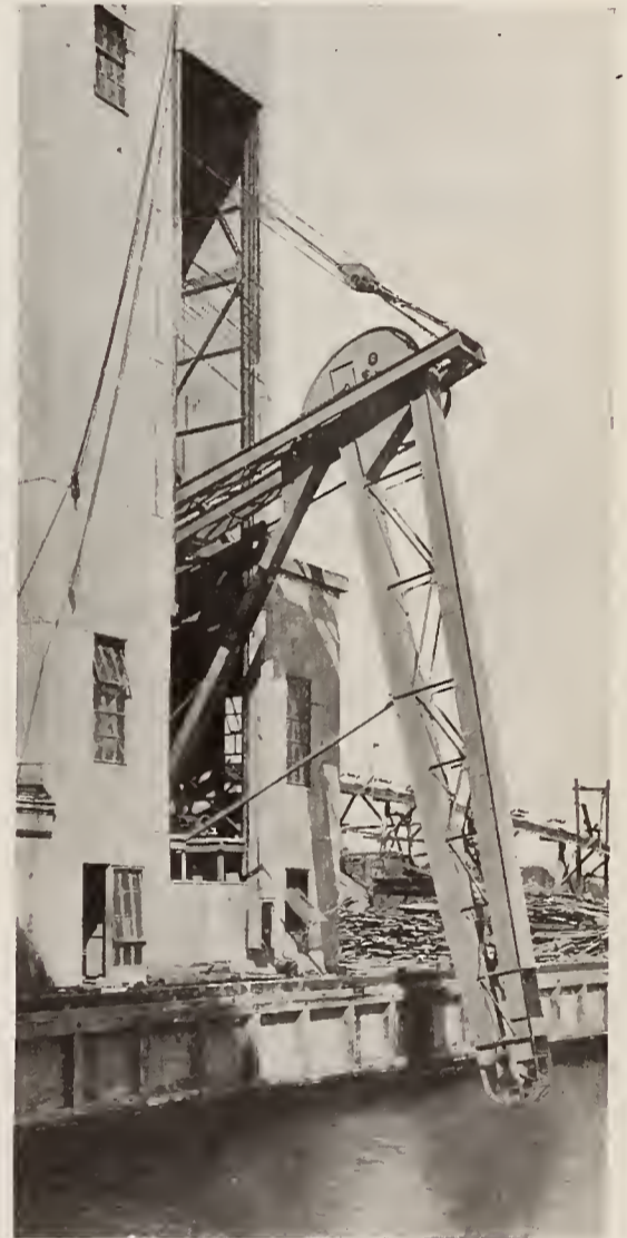
MARINE LEG NORTHERN CENTRAL ELEVATOR BALTIMORE, MD.
