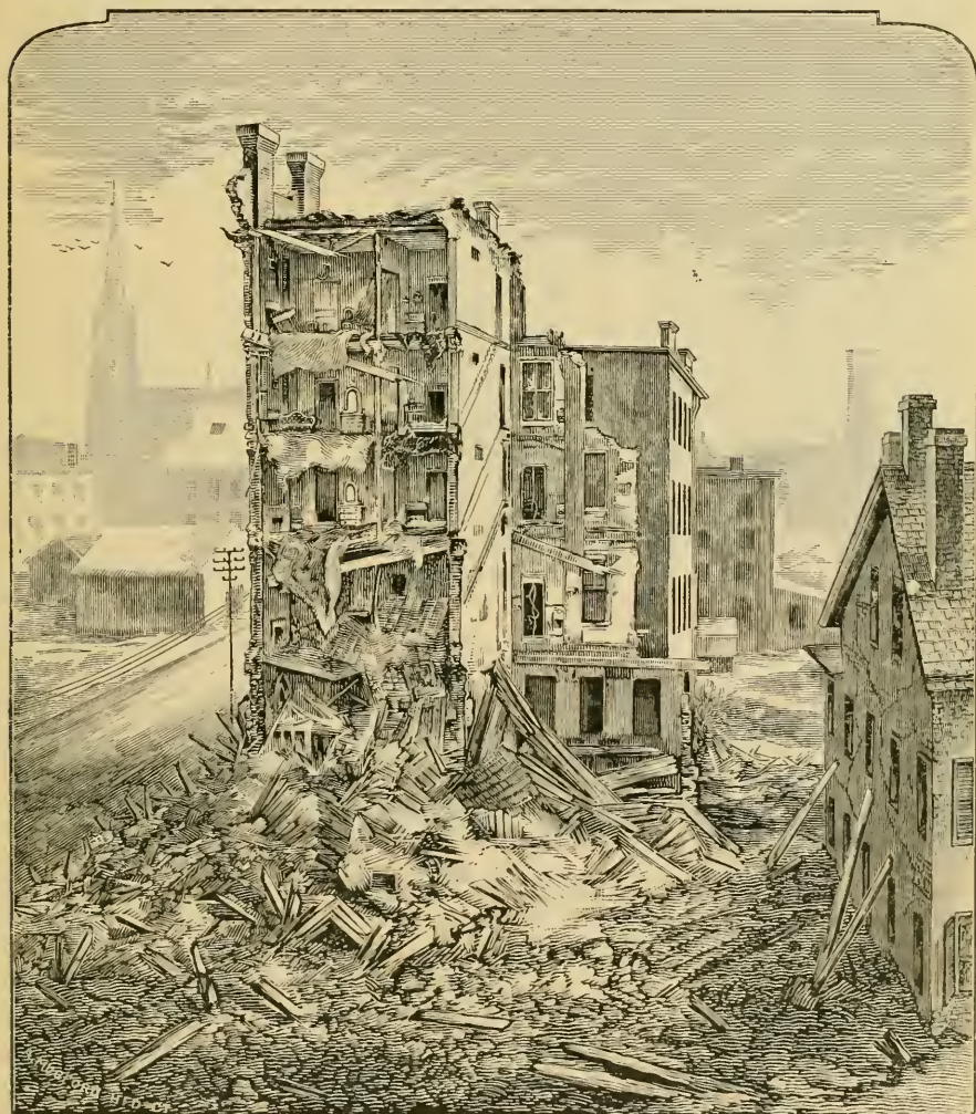
FIG. 1.—THE PARK CENTRAL HOTEL AFTER THE EXPLOSION.
