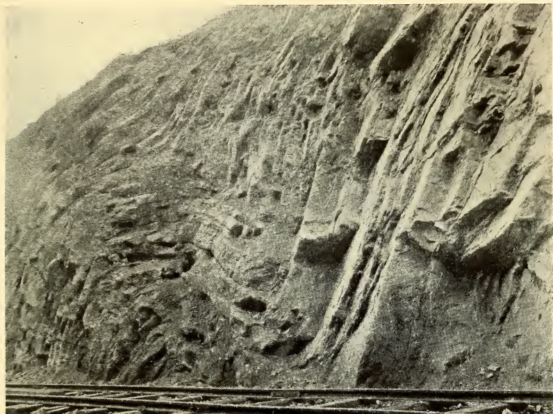
FIG. 1.—ANTICLINE AND SYNCLINE IN MOUNTAIN-LIMESTONE.
