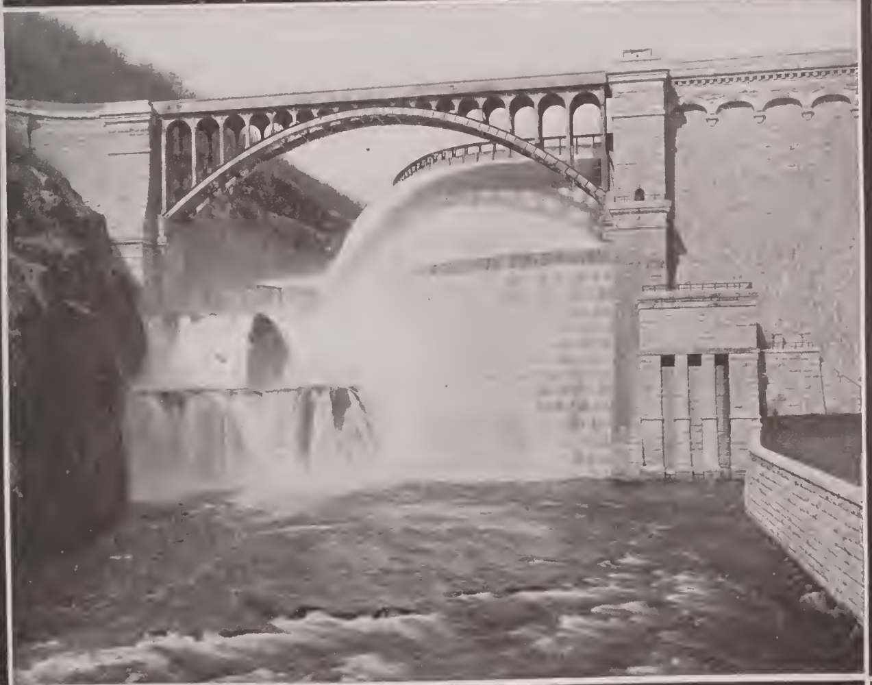
CROTON AQUEDUCT. Upper picture, main dam at Croton Falls Reservoir. Lower, new Croton Dam.
