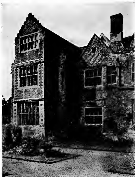
BRECCLES HALL (SOUTH-EAST GABLE).
