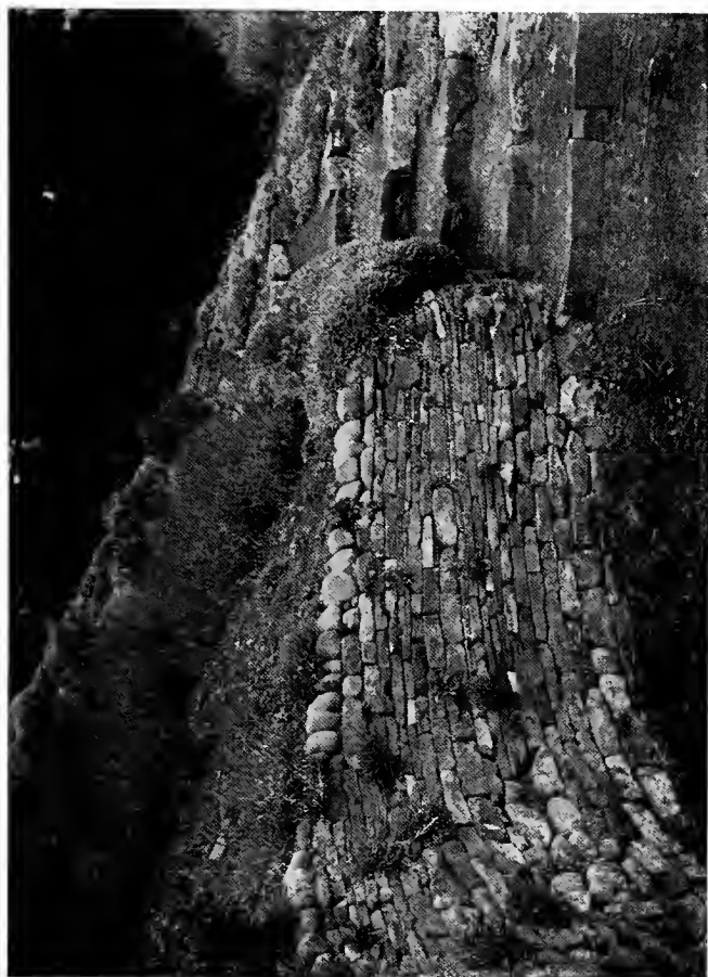
Fig. 18.—A DRY WALL SHORTLY AFTER CONSTRUCTION.
