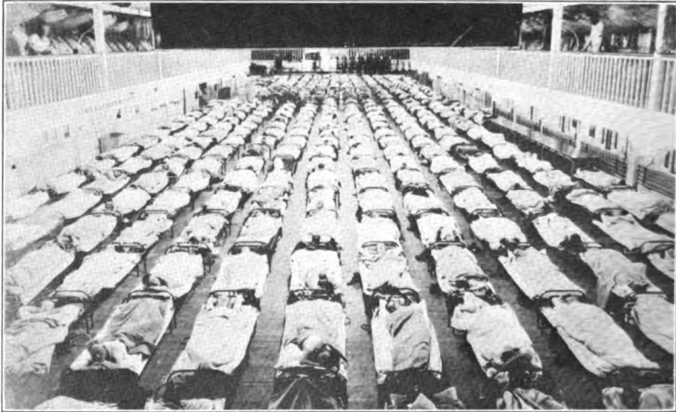
MAIN DRILL HALL AS A DORMITORY, TRAINING STATION, SAN FRANCISCO, CAL.
