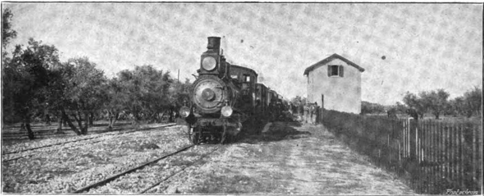
TRAIN AT LYDDA STATION.
