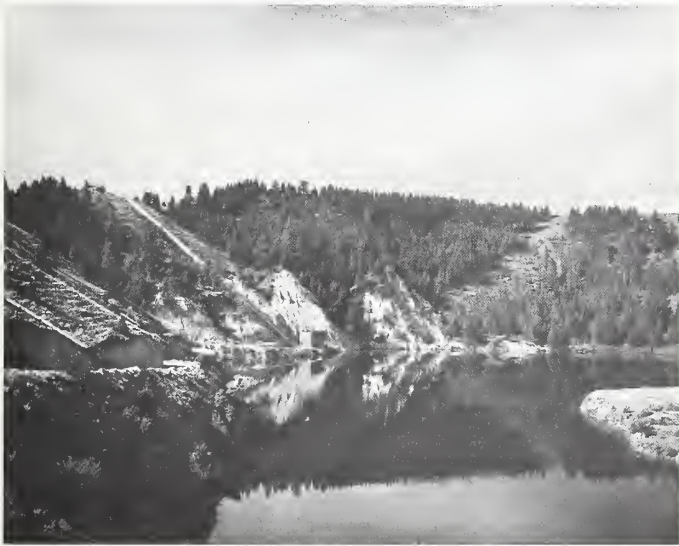
An irrigation pumping plant helps to supply the Pablo reservoir at the Flathead Reservation, Montana (Photo by Don Morrow; courtesy, Central Library, Department of the Interior).
