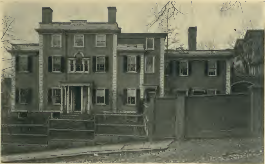
SULLIVAN DORR HOUSE, PROVIDENCE, RHODE ISLAND.
