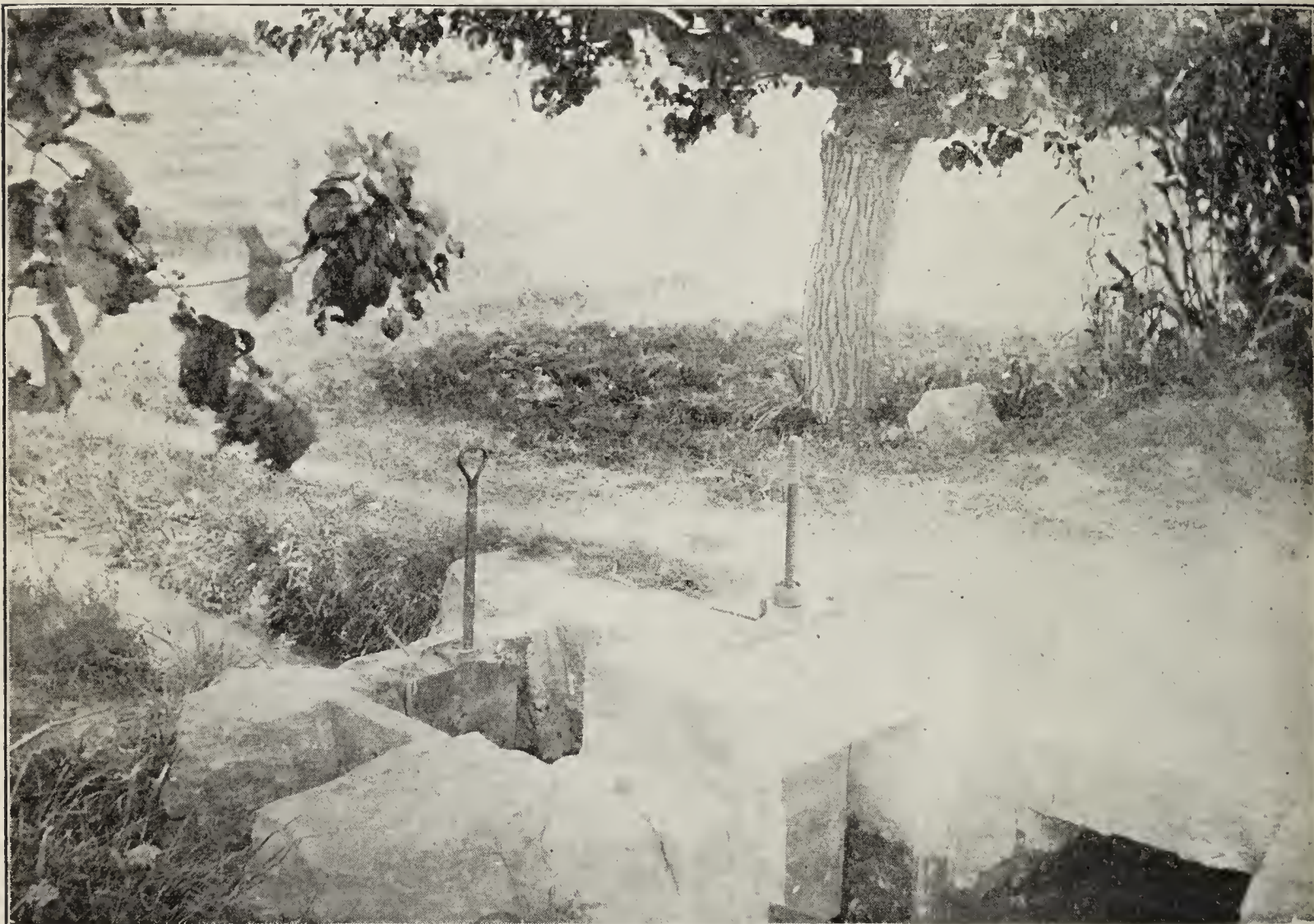
A Masonry Regulator with Iron Gates, near Arles, in Southern France.
