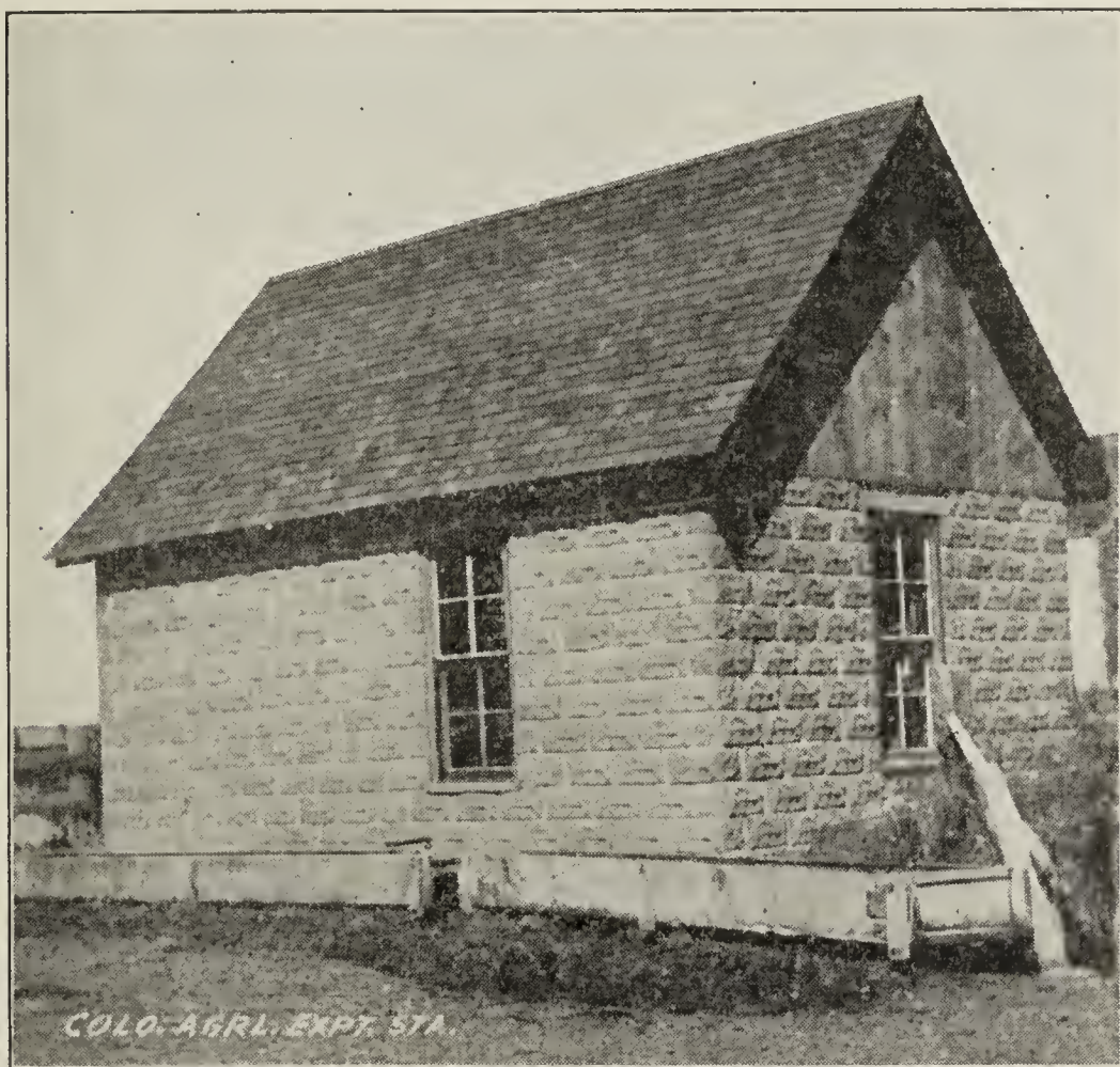
Fig 1—Cement Block Dairy.
