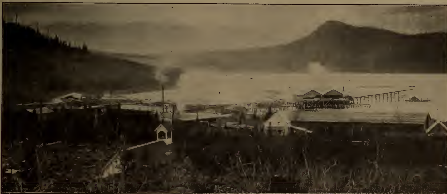
GENERAL VIEW OF SAW MILL OF CANADIAN PACIFIC LUMBER COMPANY, PORT MOODY, B. C.
