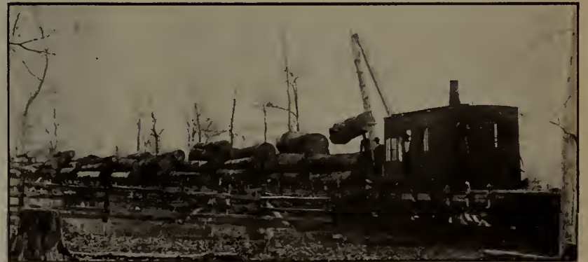
MISSISSIPPI: LOADING A TRAIN LOAD OF HEAVY LOGS WITH A "RAPID." As each load is completed the loader is slid back on to the next car (under its own power.)
