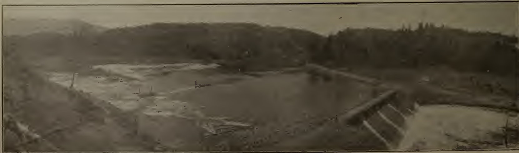
GENERAL VIEW OF DAM OF THE ST. ANNE POWER COMPANY.
