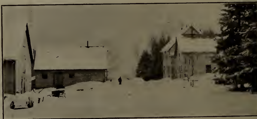
HEADQUARTERS OF THE ST. ANNE POWER COMPANY.
