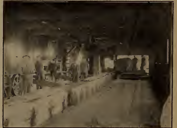
INTERIOR VIEW CAPITAL PLANING MILLS.
