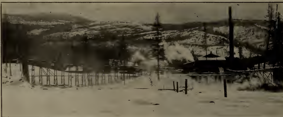
MOYIE LUMBER AND MILLING COMPANY—END VIEW OF MILL, SHOWING BOILER HOUSE, JACK LADDER, REFUSE CONVEYOR, BLOW PIPE AND PART OF MILL POND.
