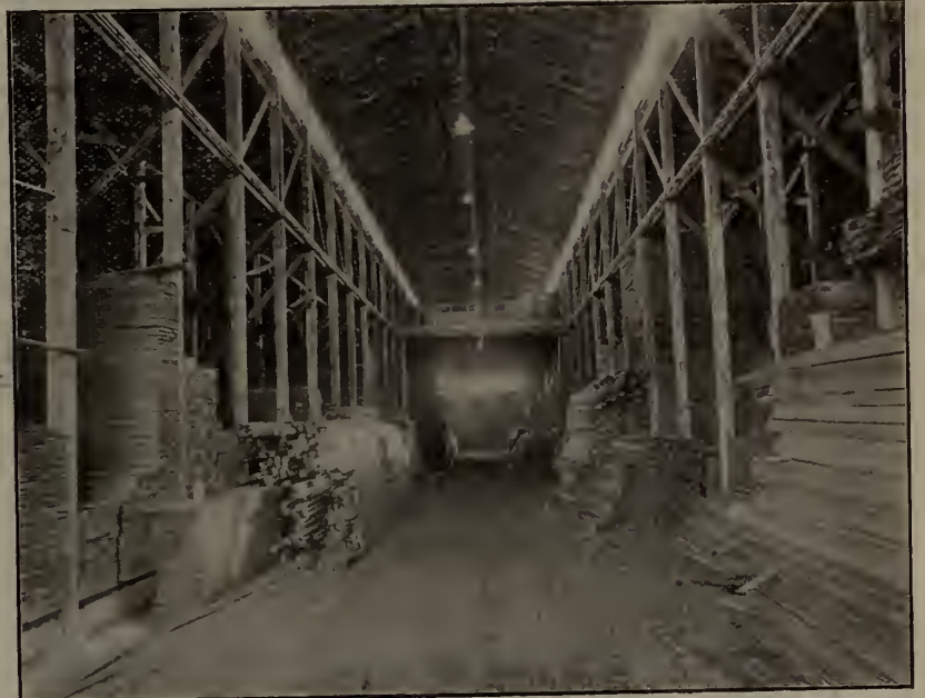
SPRAGUE LUMBER COMPANY, WINNIPEG—VIEW OF INTERIOR OF PORTION OF DRYING SHED.
