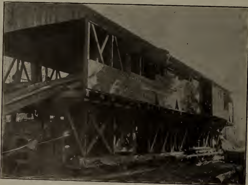
MOVABLE SAW MILL OF WILLIAM COOKE & SONS, HILLSDALE, ONT.—SIDE VIEW.
