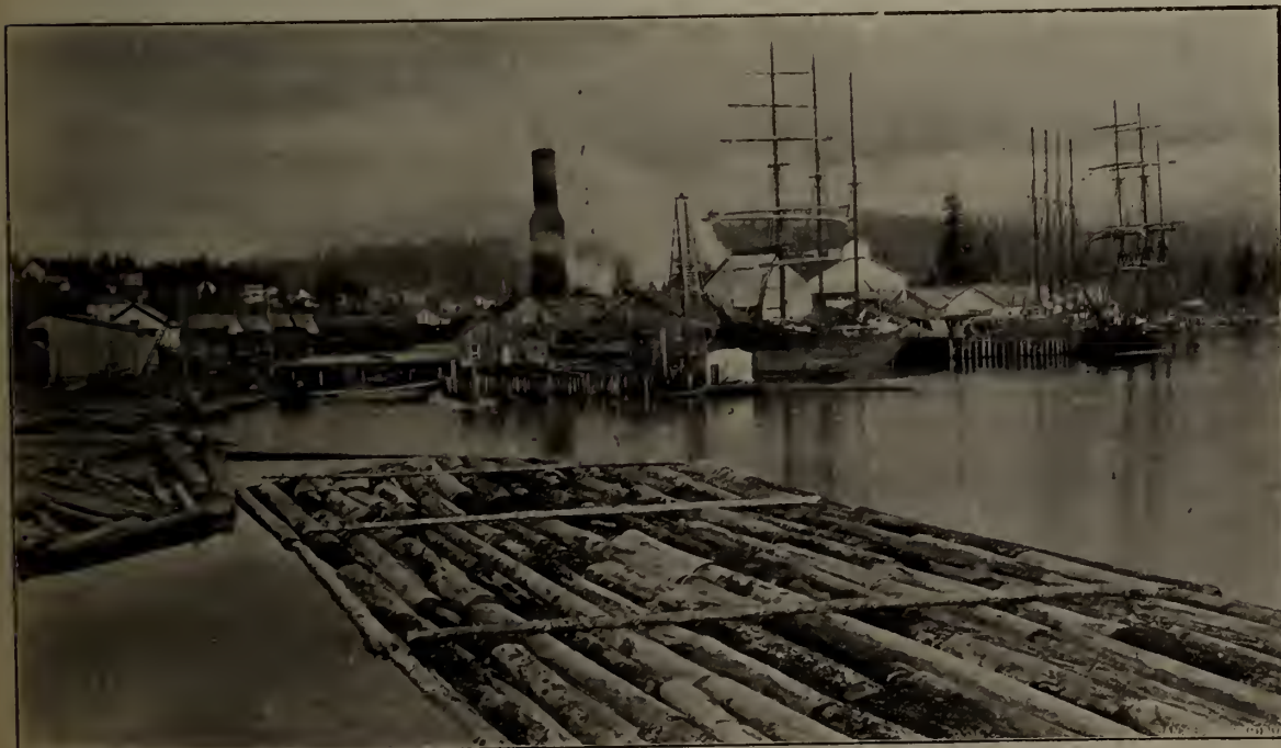
SAW MILL OF THE BRUNETTE SAWMILL COMPANY, NEW WESTMINSTER, B. C.
