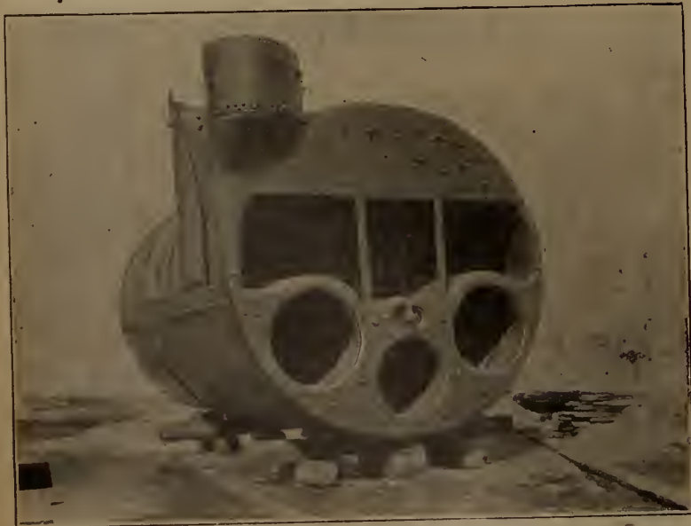
One of two Marine Boilers built in our shops for the Richelieu & Ontario Navigation Co's Steamer "Carolina." Length 21' ,diameter 13' 4", height 11' 10", weight 37 1/2 tons. }
