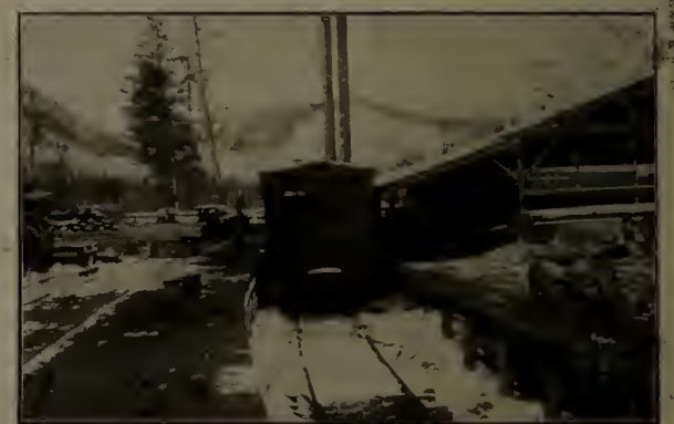
MOYIE LUMBER AND MILLING COMPANY—LOADING PLATFORMS.
