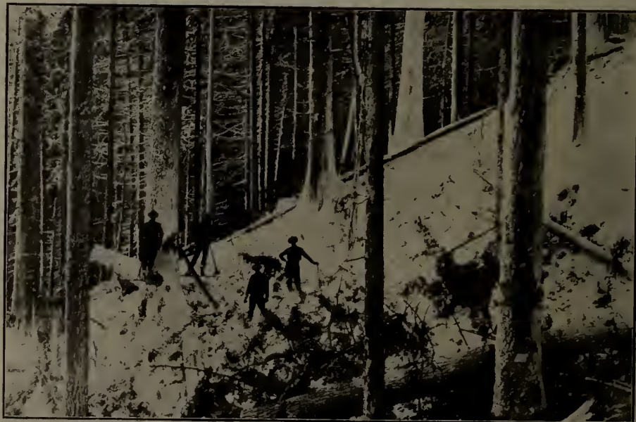
ON THE LIMITS OF THE CHEMAINUS LUMBER AND MANUFACTURING COMPANY, VANCOUVER ISLAND, B.C.
