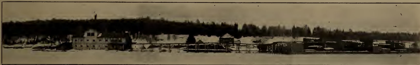
NEW MILL OF THE J. E. MURPHY LUMBER COMPANY AT MILFORD HAVEN, ONT.
