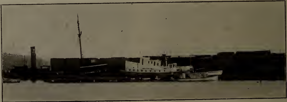
DOCKS AND LUMBER YARDS OF THE C. BECK MANUFACTURING COMPANY, PENETANGUSHENE, ONT.
