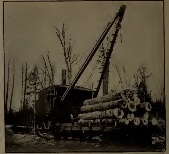
NOVA SCOTIA : THE "MCGIFFERT" LOADING LARGE LOGS AT BRIDGEWATER. After completing the first tier car is moved forward so that rear end may be loaded.
