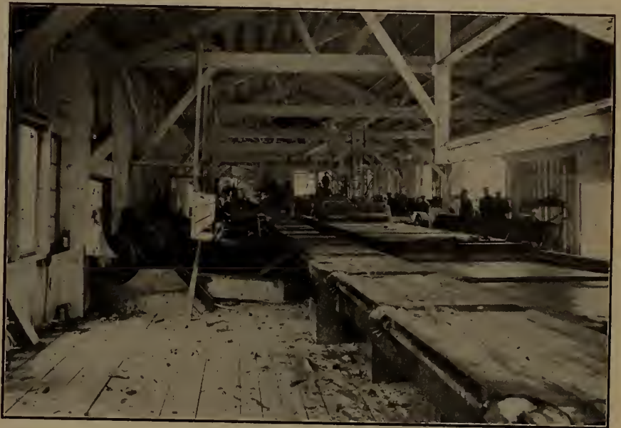
OTIS STAPLES, BAYARD, B. C.—INTERIOR VIEW OF SAW-MILL.
