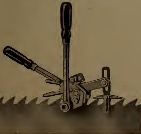
Hanchett Saw Swage for Band Saws
