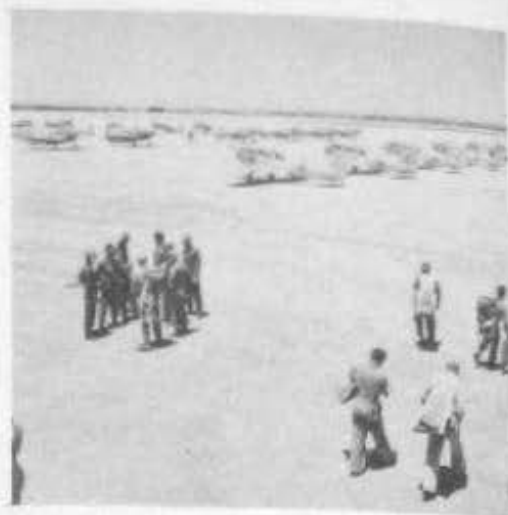
Full Gas Tanks
