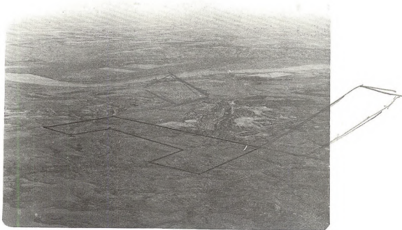
Glenharold Federal coal lease amendment (solid outline). E \frac{1}{2} E \frac{1}{2} , NW \frac{1}{4} NE \frac{1}{4} , and SW \frac{1}{4} SE \frac{1}{4} of Section 30, T. 144 N., R. 84 W., Mercer County, North Dakota. April - 1976. Aerial view looking northeast.
