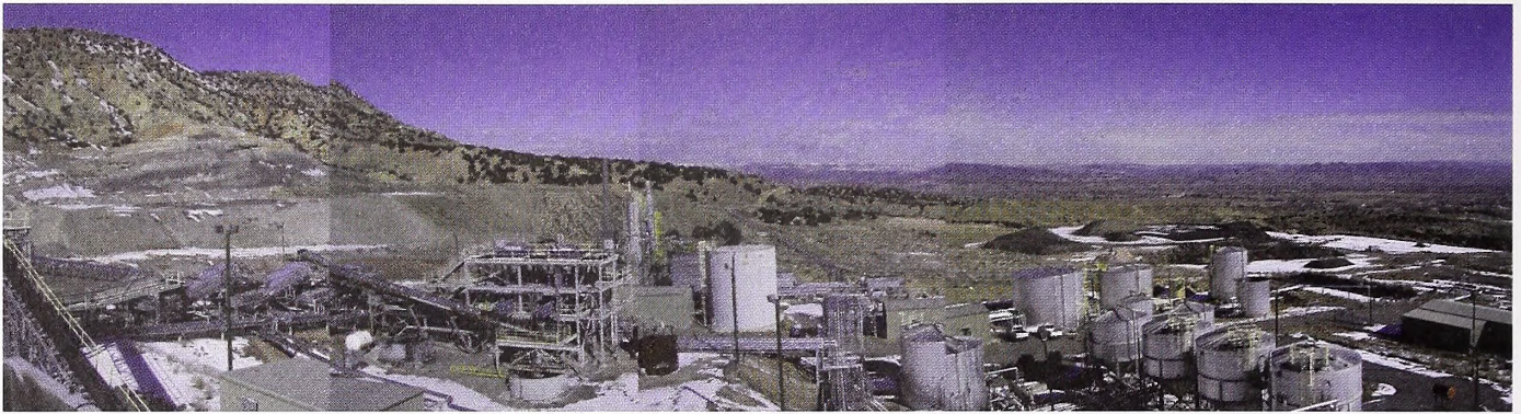
FIGURE 5.9.1-5 Photo Mosaic of Existing Pilot-Scale Tar Sands Processing Facility Utilizing Surface Mining and Solvent Extraction on Asphalt Ridge near Vernal, Utah
