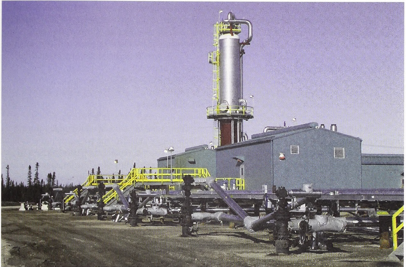
FIGURE 5.9.1-6 In Situ Steam-Assisted Gravity Drainage (SAGD) Facility near Fort McMurray, Alberta, Canada (SAGD technology uses underground wells to inject steam into the oil sands deposits and collect the bitumen released by the heat.) (Image courtesy of Suncor Energy, Inc.)
