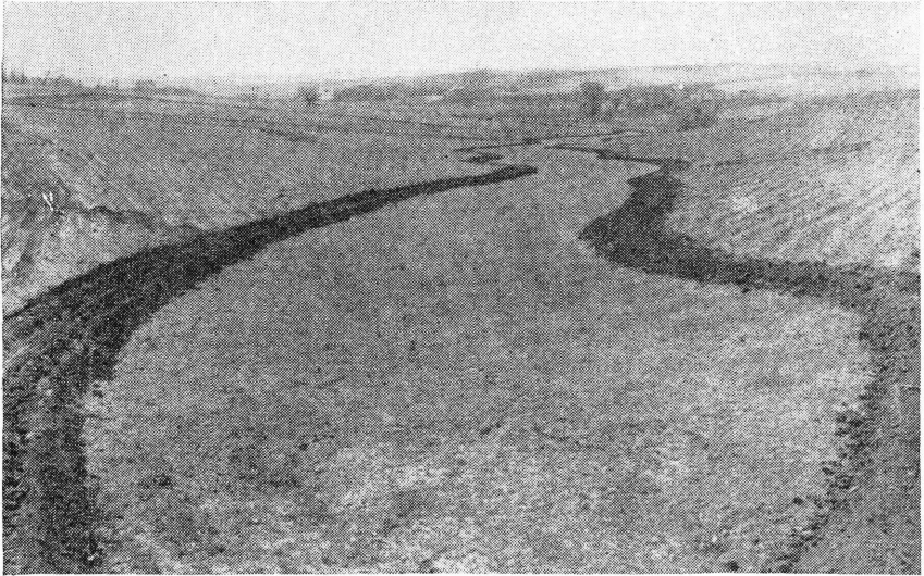
FIGURE 15.—Ridges along the sides protect newly seeded meadow outlet. Terraces will be constructed when the sod is well established.
