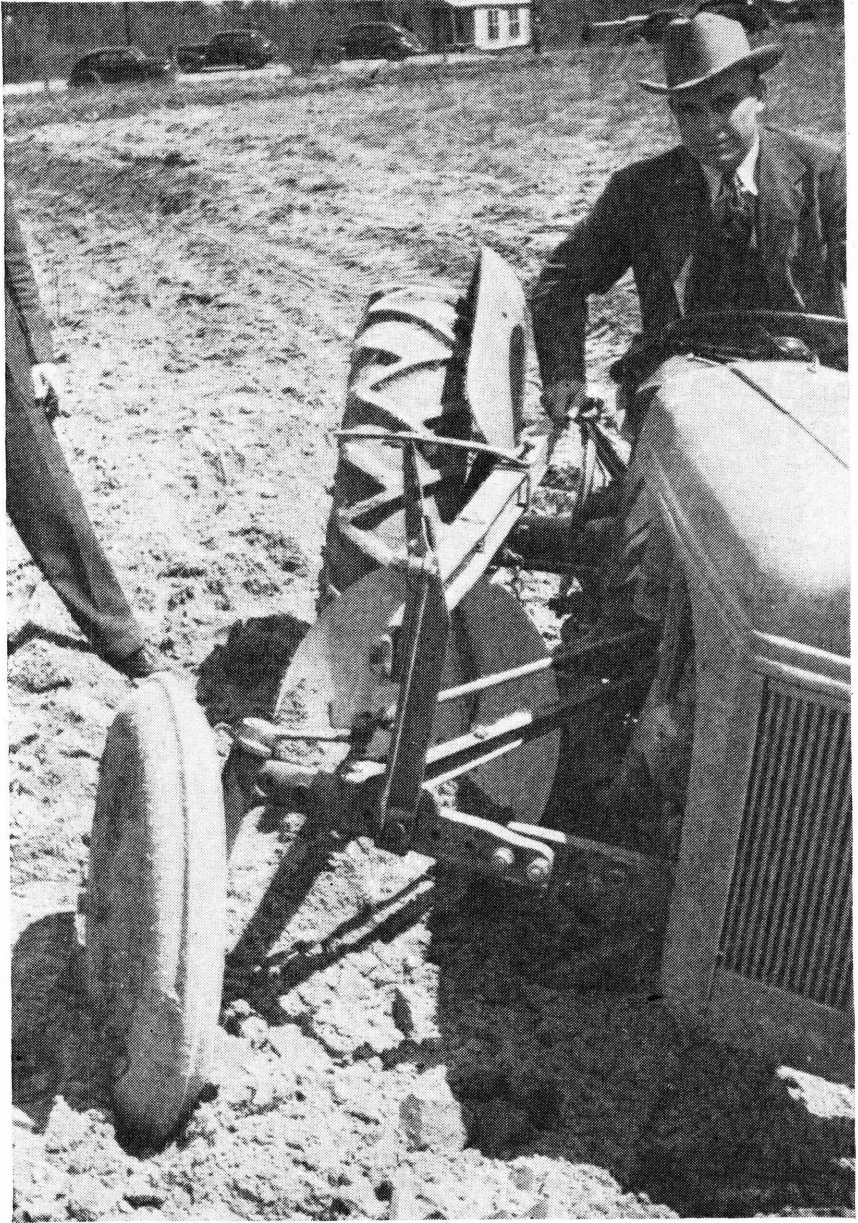
FIGURE 31.—A special disk attachment for farm tractors has proved efficient for terrace construction.
