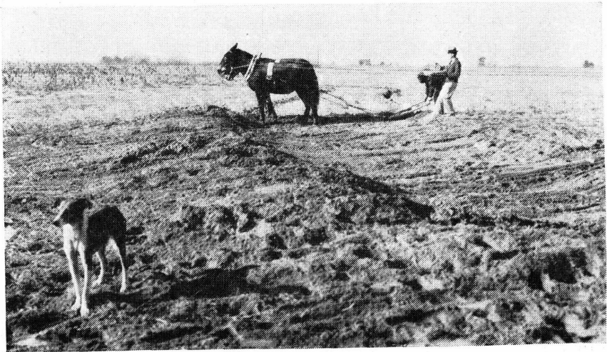
FIGURE 26.—Building a channel terrace with a slip scraper.
