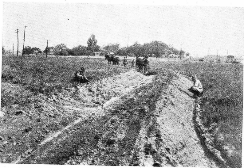
FIGURE 24.—Terrace construction with a plow and V-drag. It requires considerable work to construct satisfactory terraces with this type of equipment.
