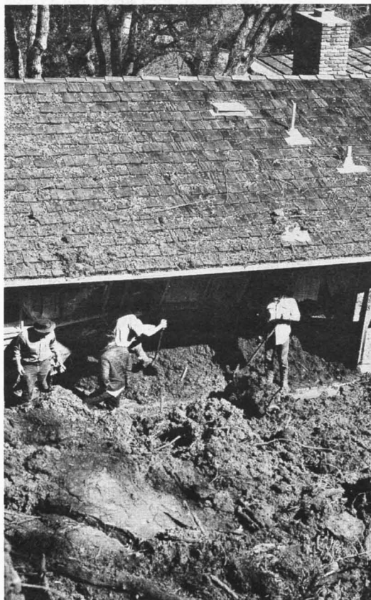
Soil saturated with water slides down steep slope, damaging home.
