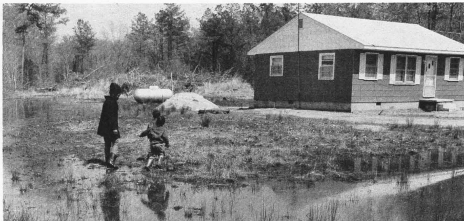
This site appeared desirable when home was built during dry season. Soil survey would have indicated extreme wetness after heavy rains or spring thaw.
