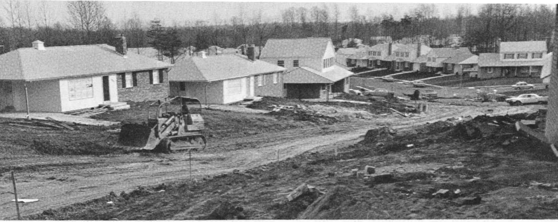
Construction of new homes near Largo, Md., a suburb of Washington.
