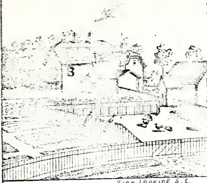
View Looking S.E.
