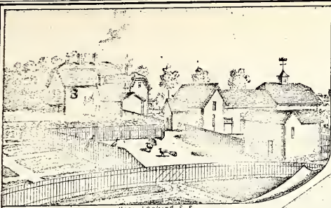
View Looking S.E.
