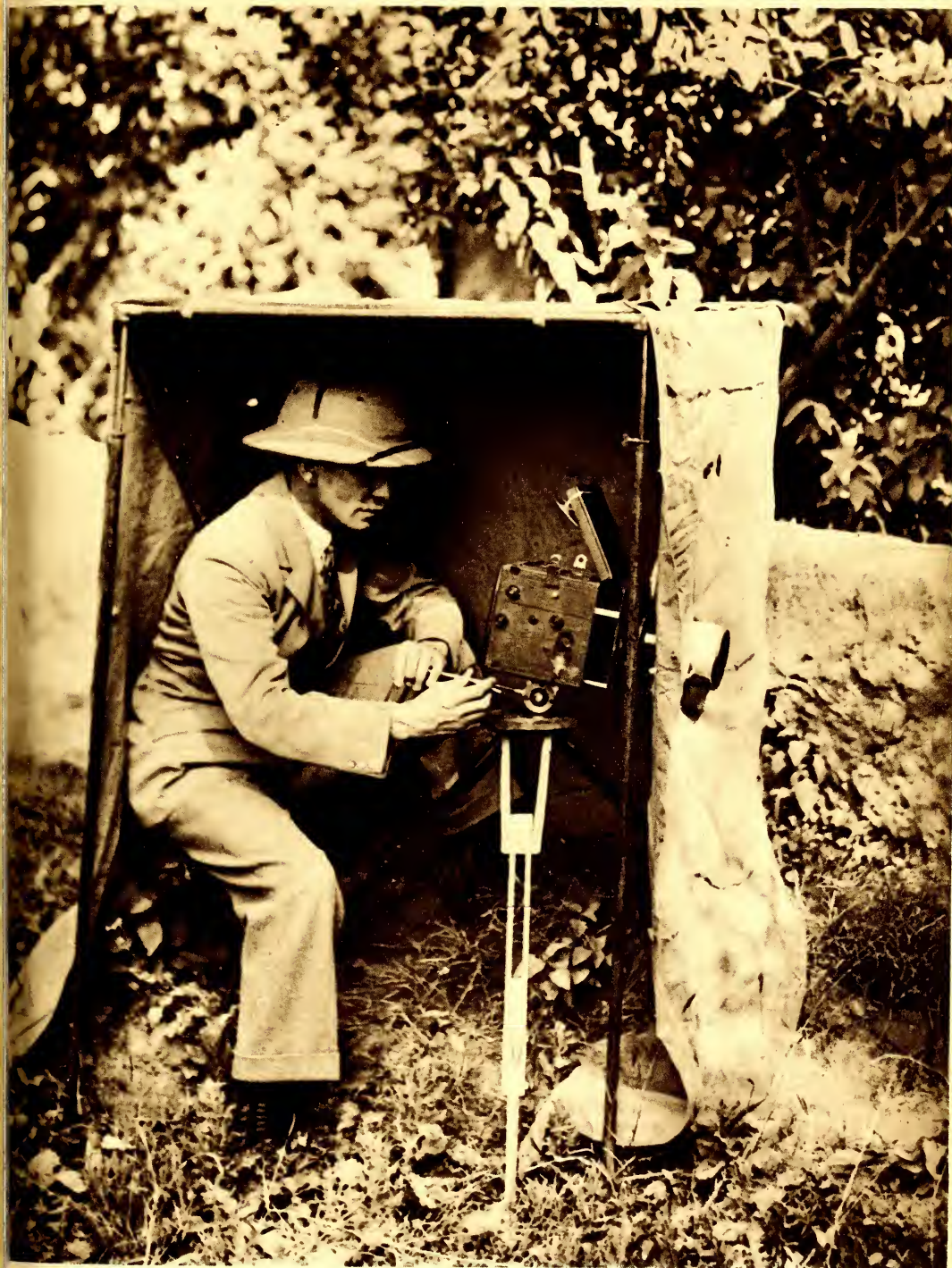
The Hide, uncamouflaged and with one side raised to show its construction. It is pitched on a sloping bank.
